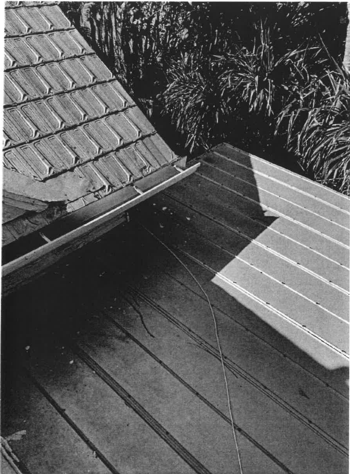
Photo of property under review. View of front elevation showing 5 v-crimp on lower addition.
