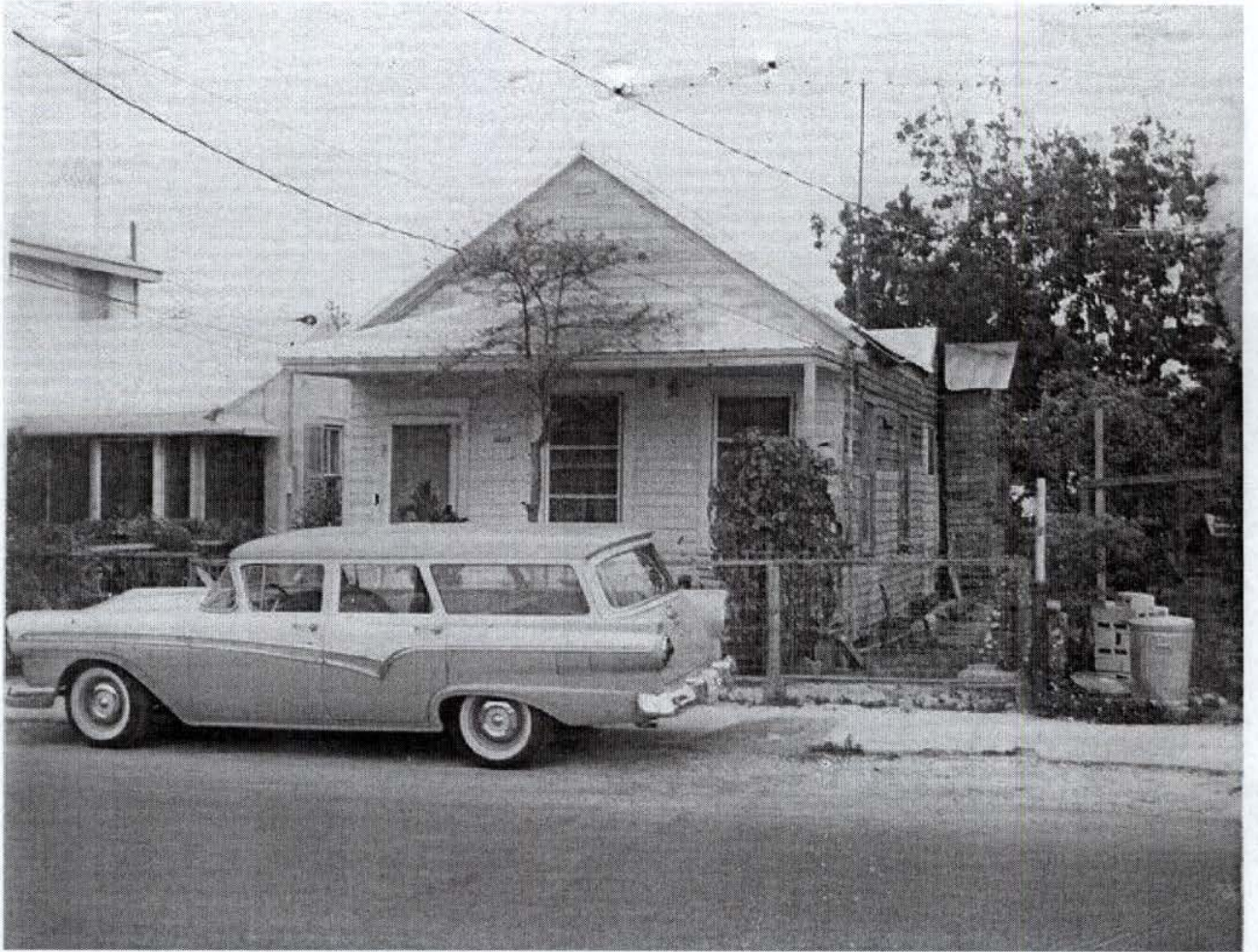
Photo taken by the Property Appraiser's office c1965; 1107 Virginia St.; Tract 13, Monroe County Library
