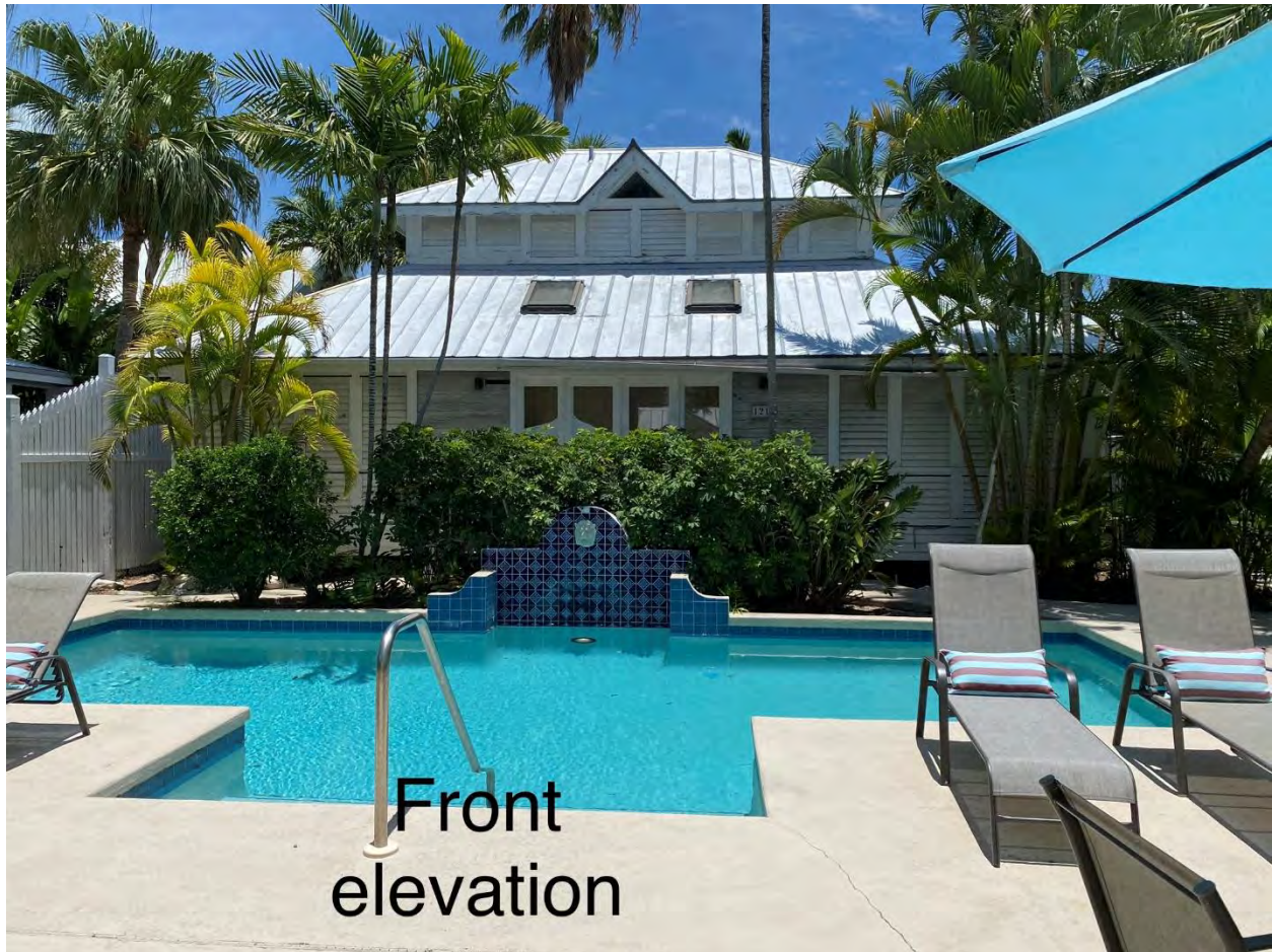
Photograph of the house front elevation.
