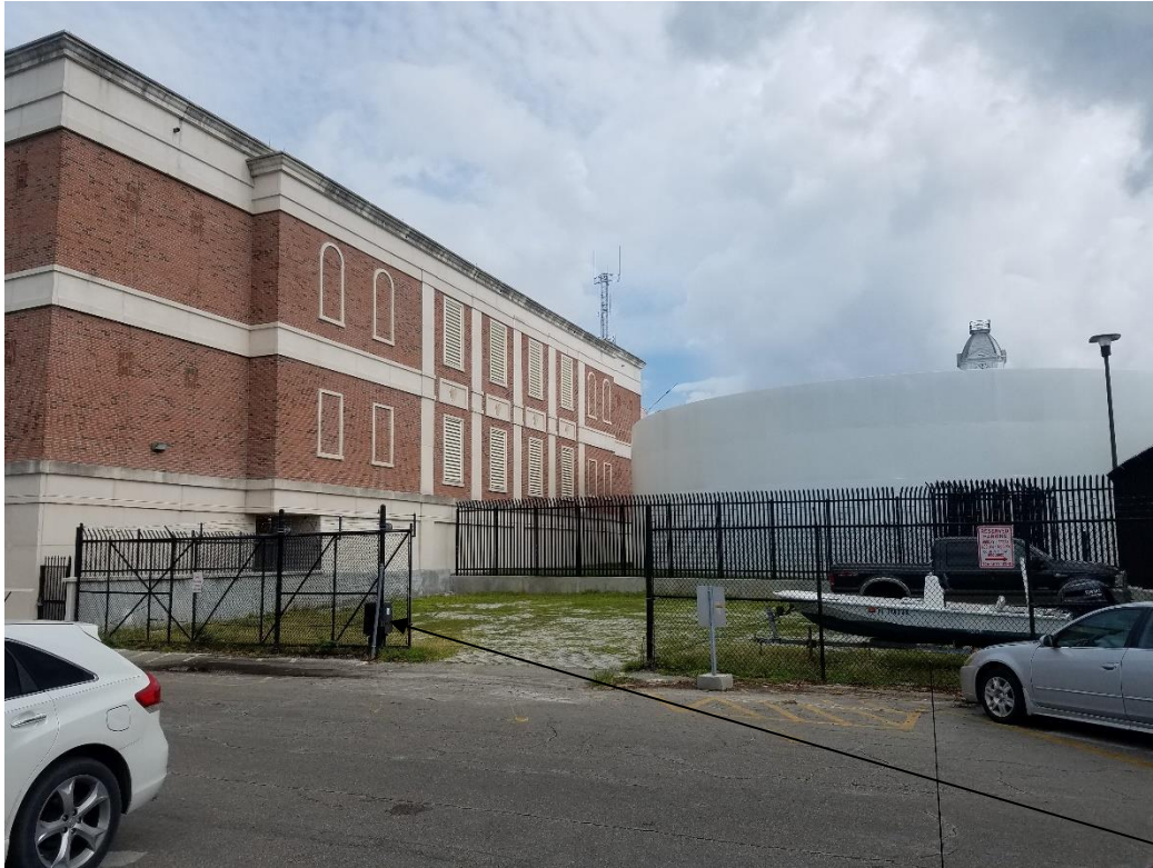
Street view of lot where proposed Chiller Plant is being constructed. Building to be constructed here.
