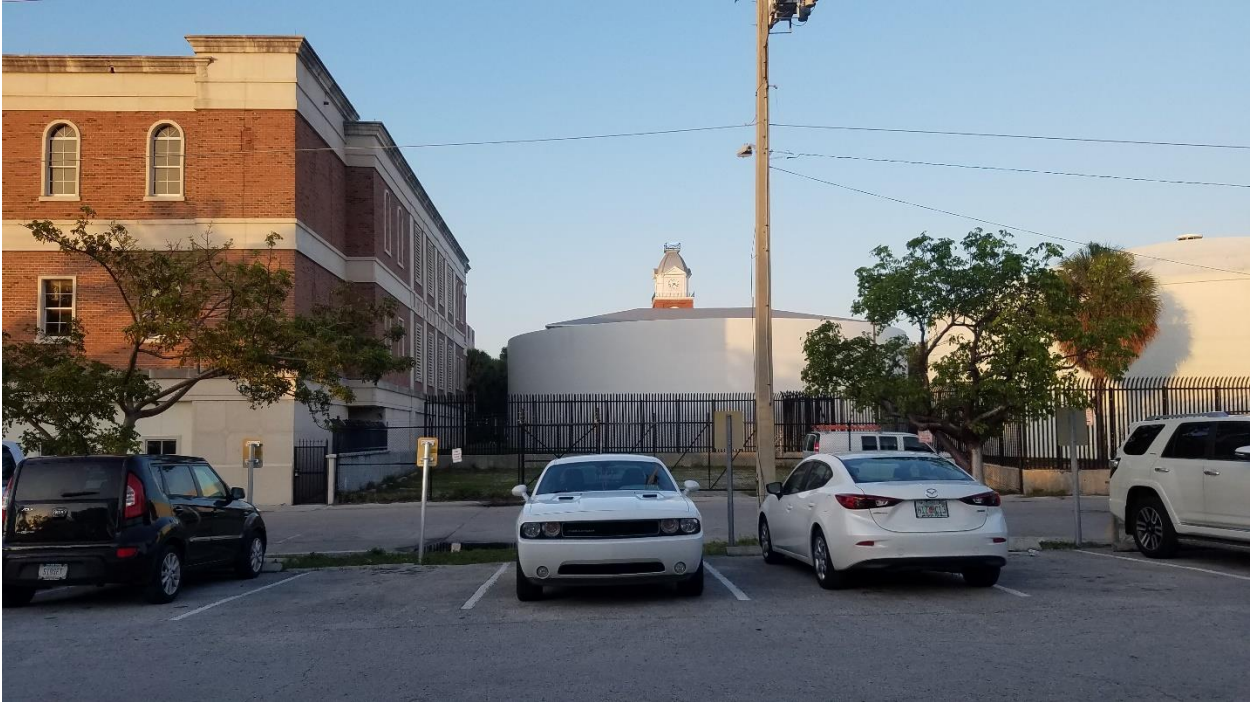
Adjacent building: A large FKAA water tank is located to the right of the site, as well as behind the site.
