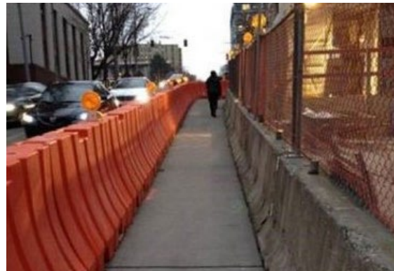
Pedestrian route adjacent to construction
