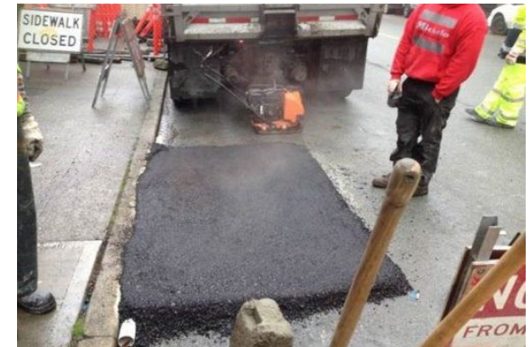
Temporary curb ramp along pedestrian detour
