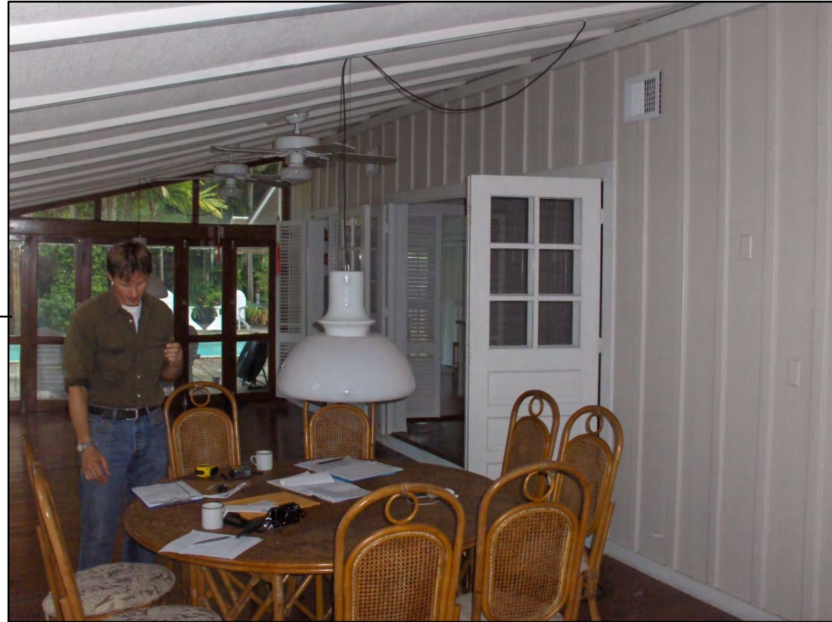
PHOTOGRAPH SHOWING THE BOARD & BATTEN AT HISTORIC STRUCTURE (NORTH SIDE)
