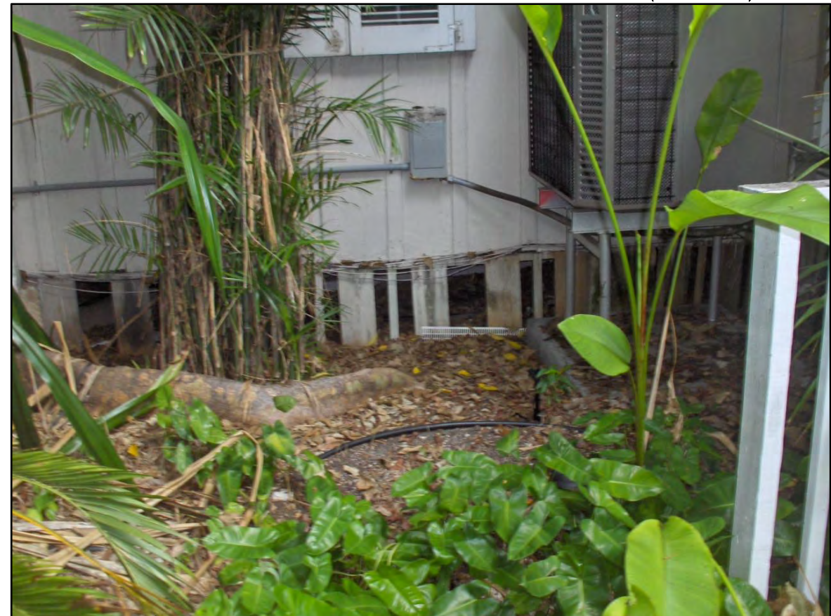
DETAIL PHOTOGRAPH SHOWING THE BOARD AND BATTEN AT HISTORIC STRUCTURE (SOUTH SIDE)
