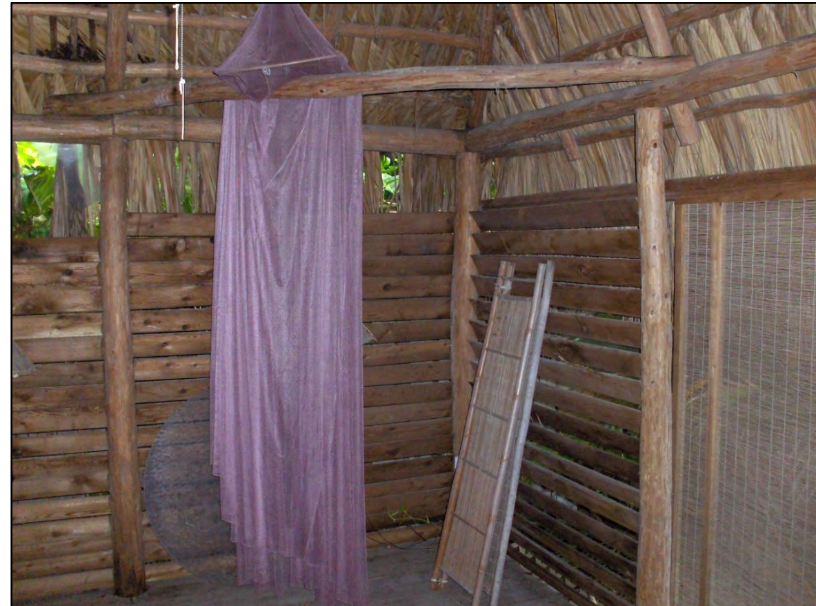
PHOTOGRAPH OF THE INTERIOR OF THE ACCESSORY STRUCTURE
