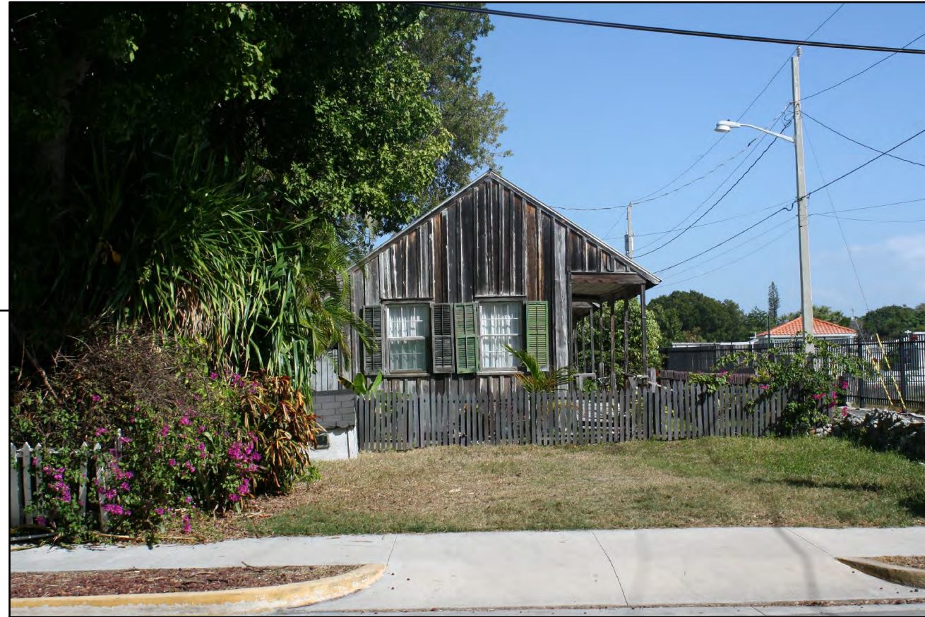
PHOTOGRAPH OF ADJACENT PROPERTY TO THE SOUTH
