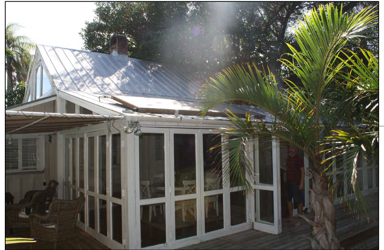
PHOTOGRAPH OF THE ADDITION TO THE NORTH OF THE HISTORIC STRUCTURE FROM THE SIDE YARD
