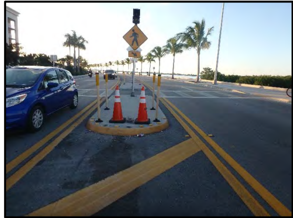
Photo 1: Looking east along US 1 at Crosswalk 1.
