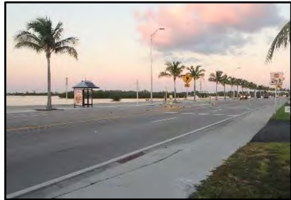
Photo 5: Looking east at Crosswalk 2.
