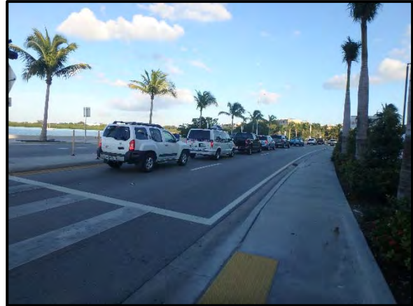
Photo 4: Looking east along US 1 at Crosswalk 1. Note the eastbound traffic queues from the downstream signal that were observed to extend up to Crosswalk 1.
