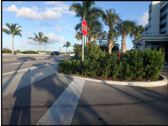
Photo 3: Looking east from the driveway west of Crosswalk 1. Note the sight obstruction by trees/shrubs at the driveway.
