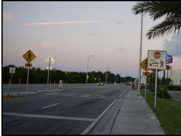
Photo 9: Looking east at Crosswalk 4.
