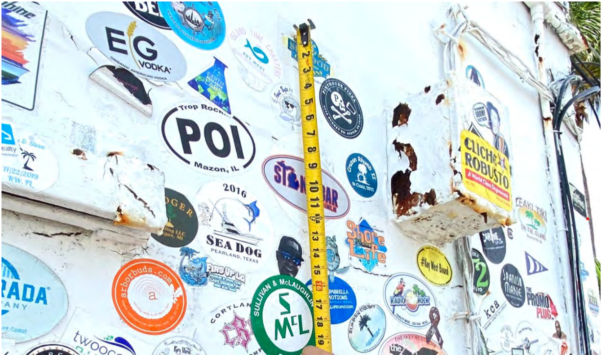
Figure 8. Partial Front elevation. Cracks outside on the tie-beam. Please note that exterior cracks were patched with stucco over time and are not as obvious.
