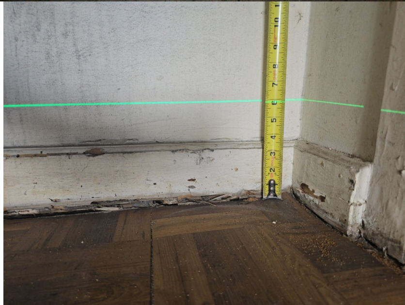
UNLEVEL FLOOR (SUNKEN FOUNDATION & FRAMING)
