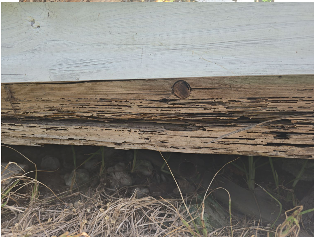
DETERIORATED RIM JOIST
