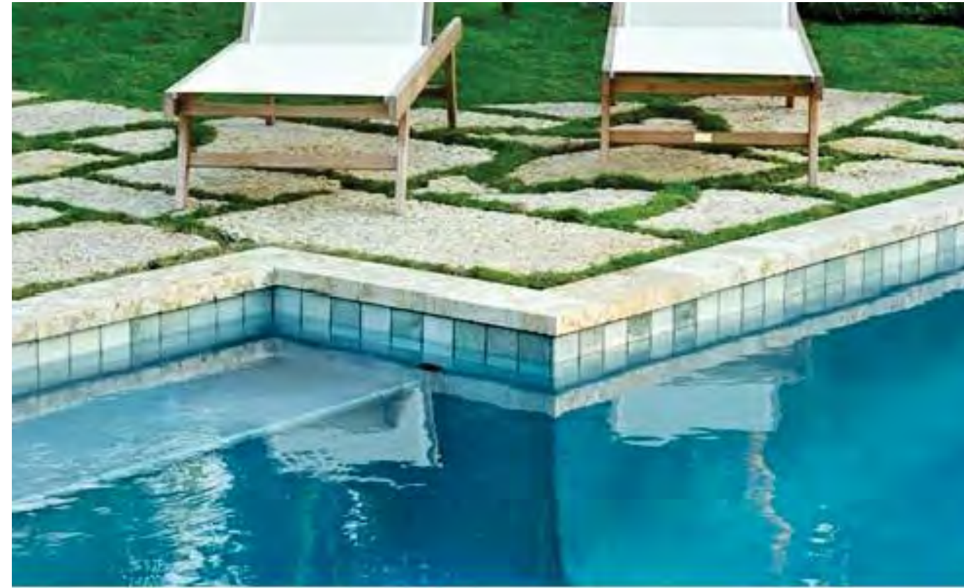
CORAL-STONE SWIMMING POOL AND SPA COPING WITH NATURAL STONE WATERLINE TILE AND STEEL BLUE POOL FINISH
