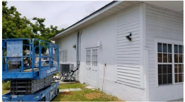
Subject Exterior – office building
