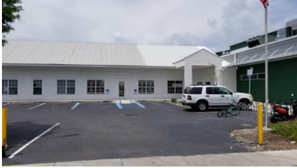
Subject Exterior – office building
