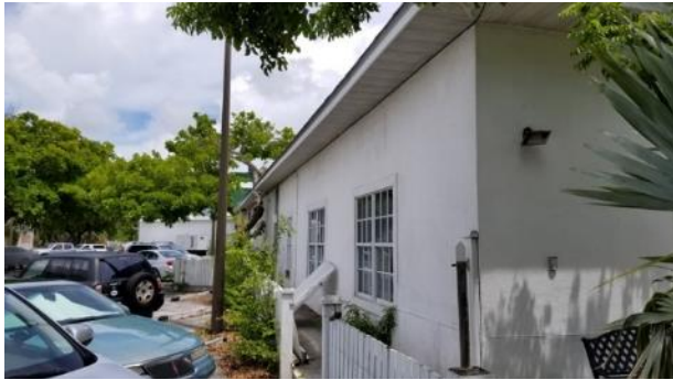
Subject Exterior – office building
