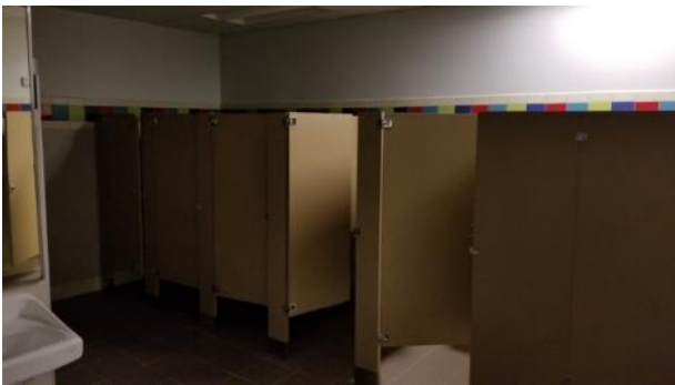
Interior of renovated gym – restroom
