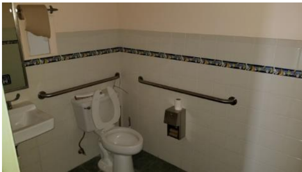
Interior of office space – single story building
