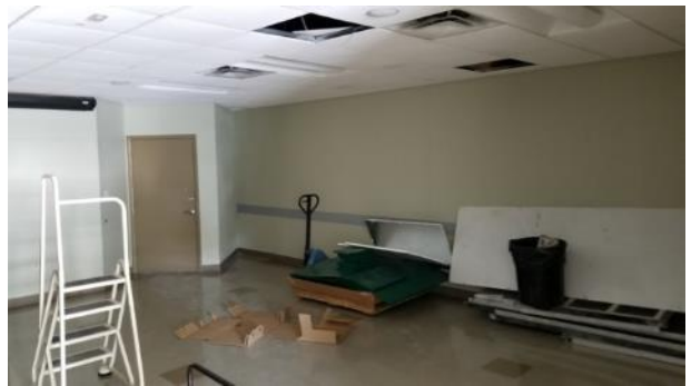
Interior of office space – single story building
