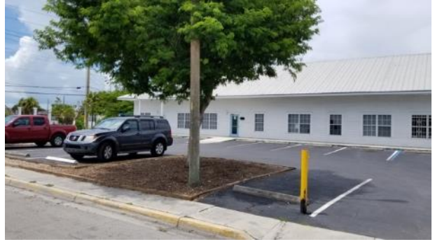
Subject Exterior – office building
