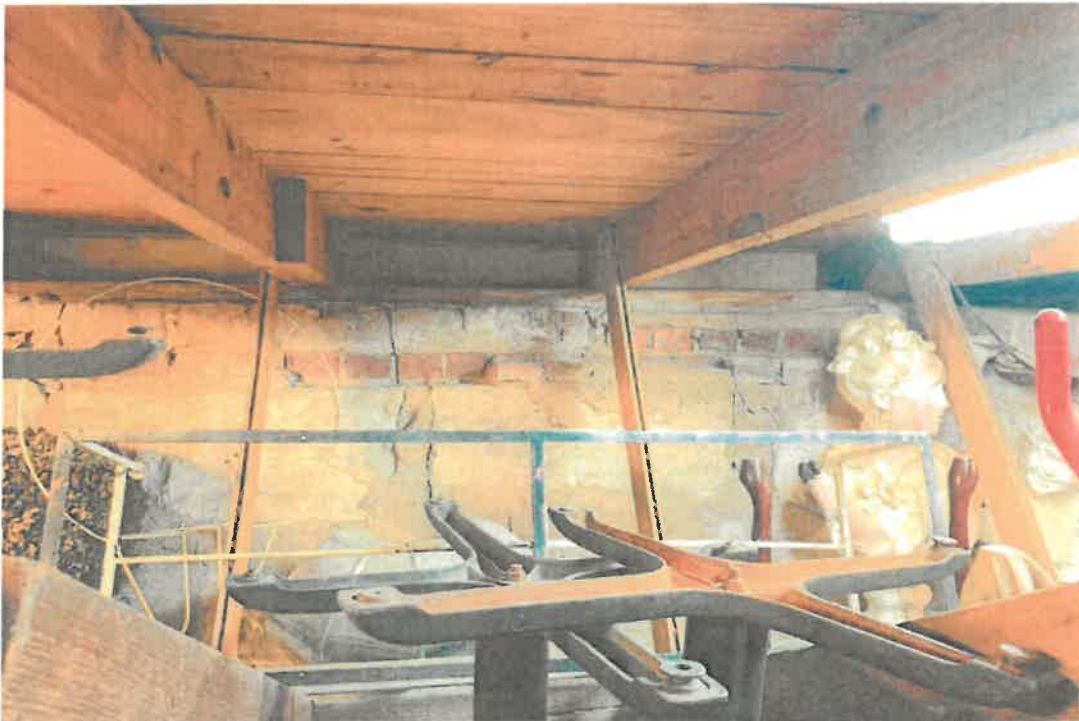
58. Tift and Mallory Warehouse / Waterfront Playhouse, attic, camera facing west. Note cracks in top of wall and below roof framing.
