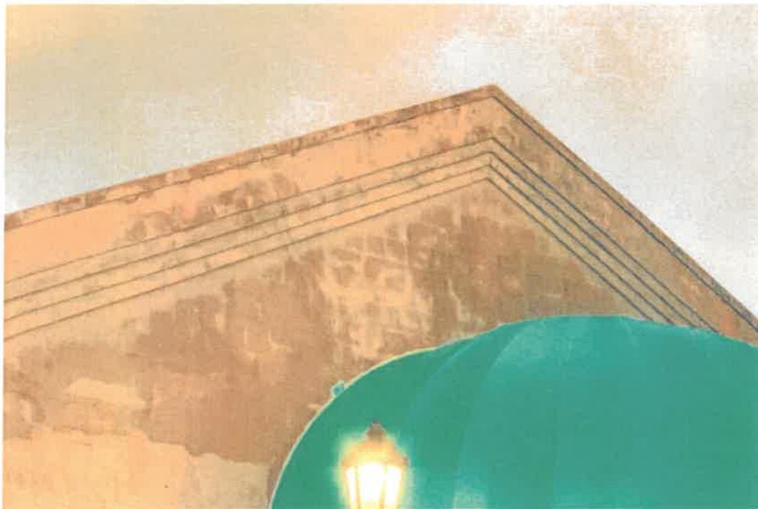
50. Tift and Mallory Warehouse / Waterfront Playhouse, partial east elevation, camera facing northwest. Note saturation of parge coat and cracking.
