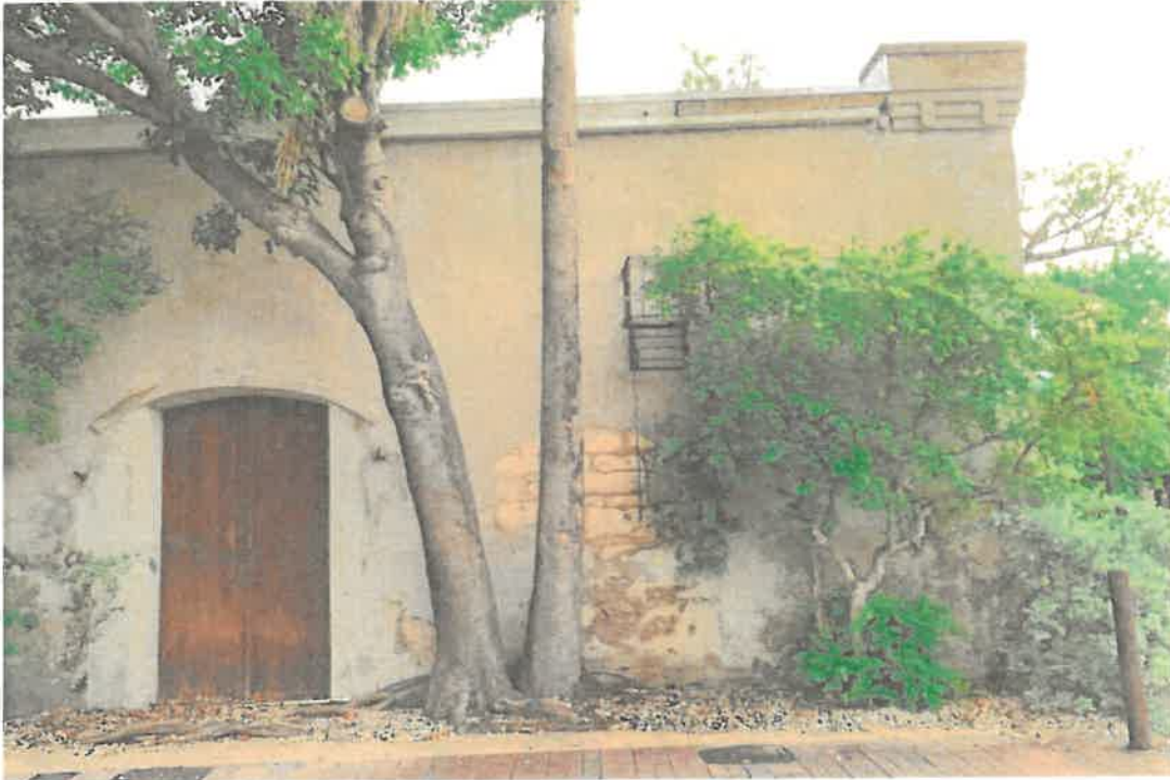
55. Tift and Mallory Warehouse / Waterfront Playhouse, partial south elevation. Note deteriorated parge coat and cracking.
