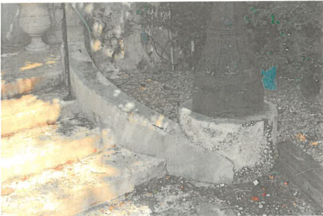
53. Tift and Mallory Warehouse / Waterfront Playhouse, front entry steps at east elevation, camera facing down and northwest. Note deterioration of steps.
