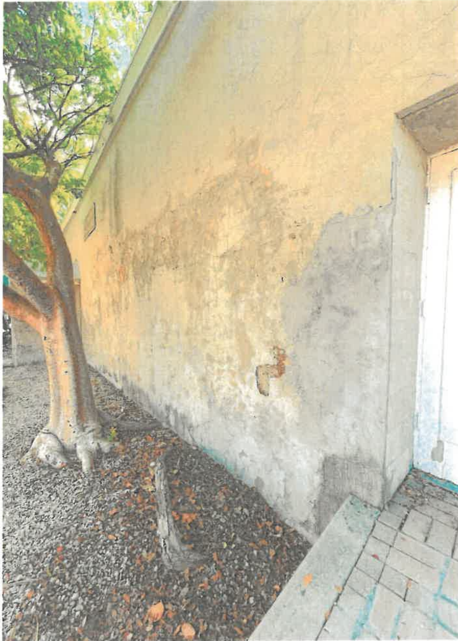
56. Tift and Mallory Warehouse / Waterfront Playhouse, partial west elevation. Note severe deterioration and failure of parge coat.
