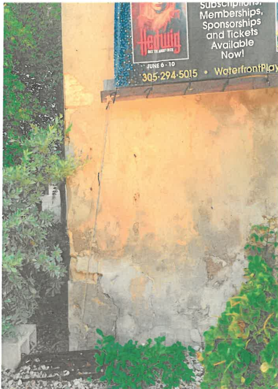
51. Tift and Mallory Warehouse / Waterfront Playhouse, partial east elevation, camera facing west. Note deterioration of parge coat and limestone.
