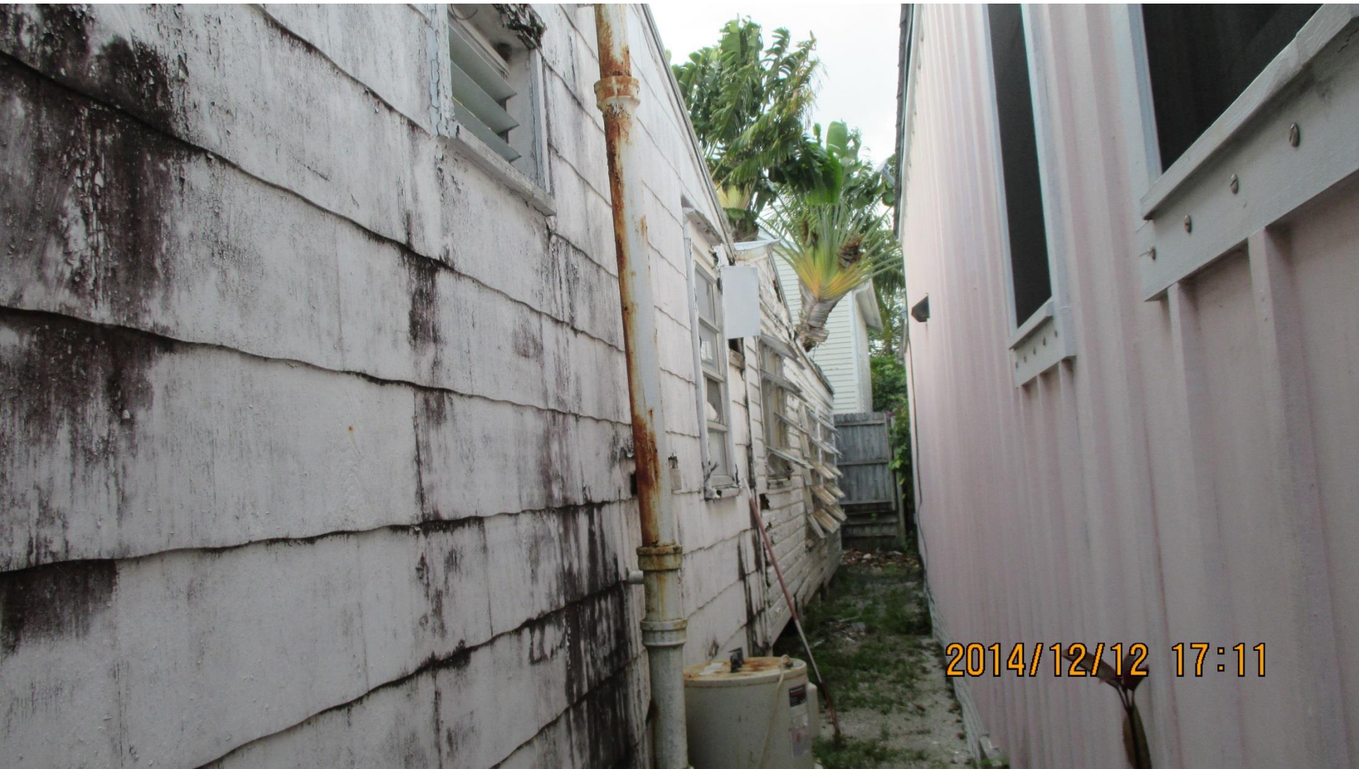
Asbestos siding on the main house and the shed roof addition. Novelty siding on the other rear additions. Note the board and batten siding on the neighboring house at 1311 Newton.
