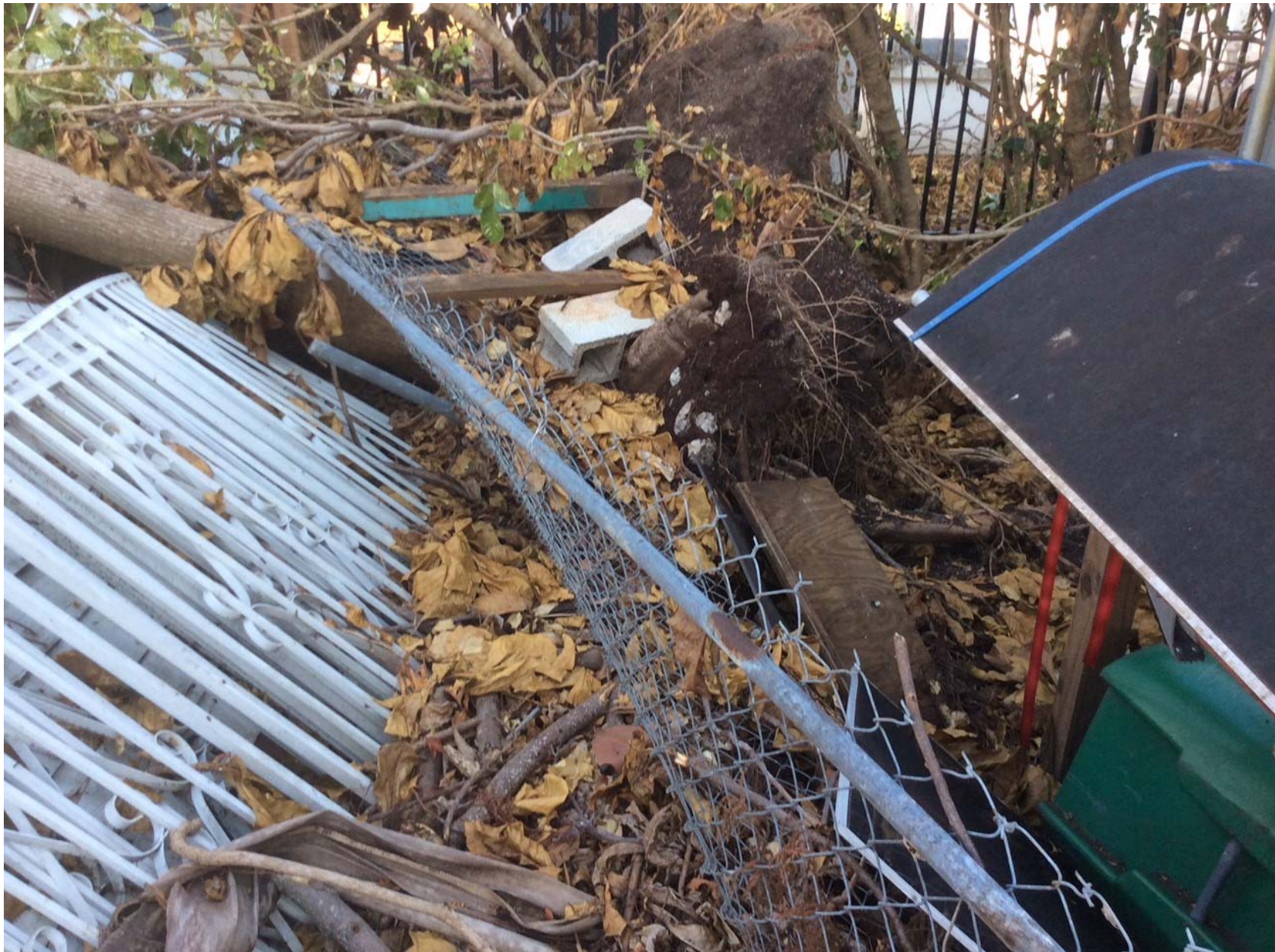
805 Olivia Street, Key West, Florida 33040 HURRICANE IRMA DAMAGE TO EXISTING NON-CONFORMING STRUCTURE
