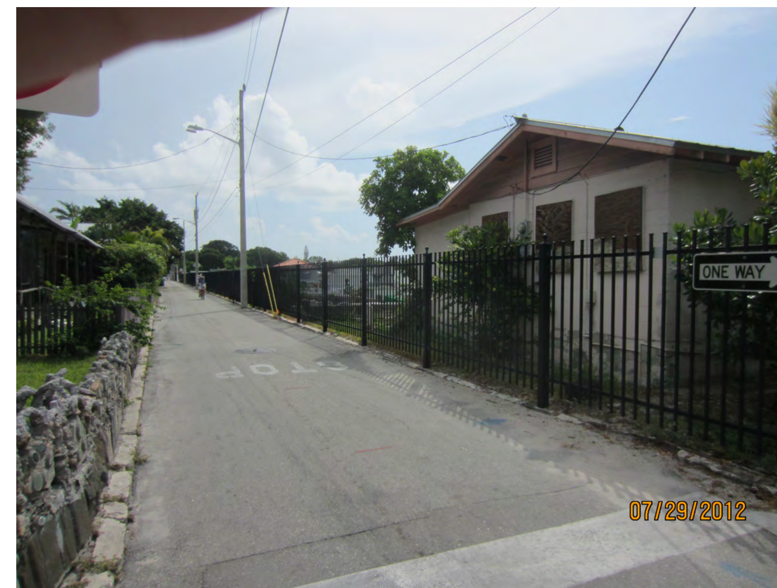
NORTH SIDE OF EXISTING SEXTON'S HOUSE LOOKING UP ANGELA STREET
