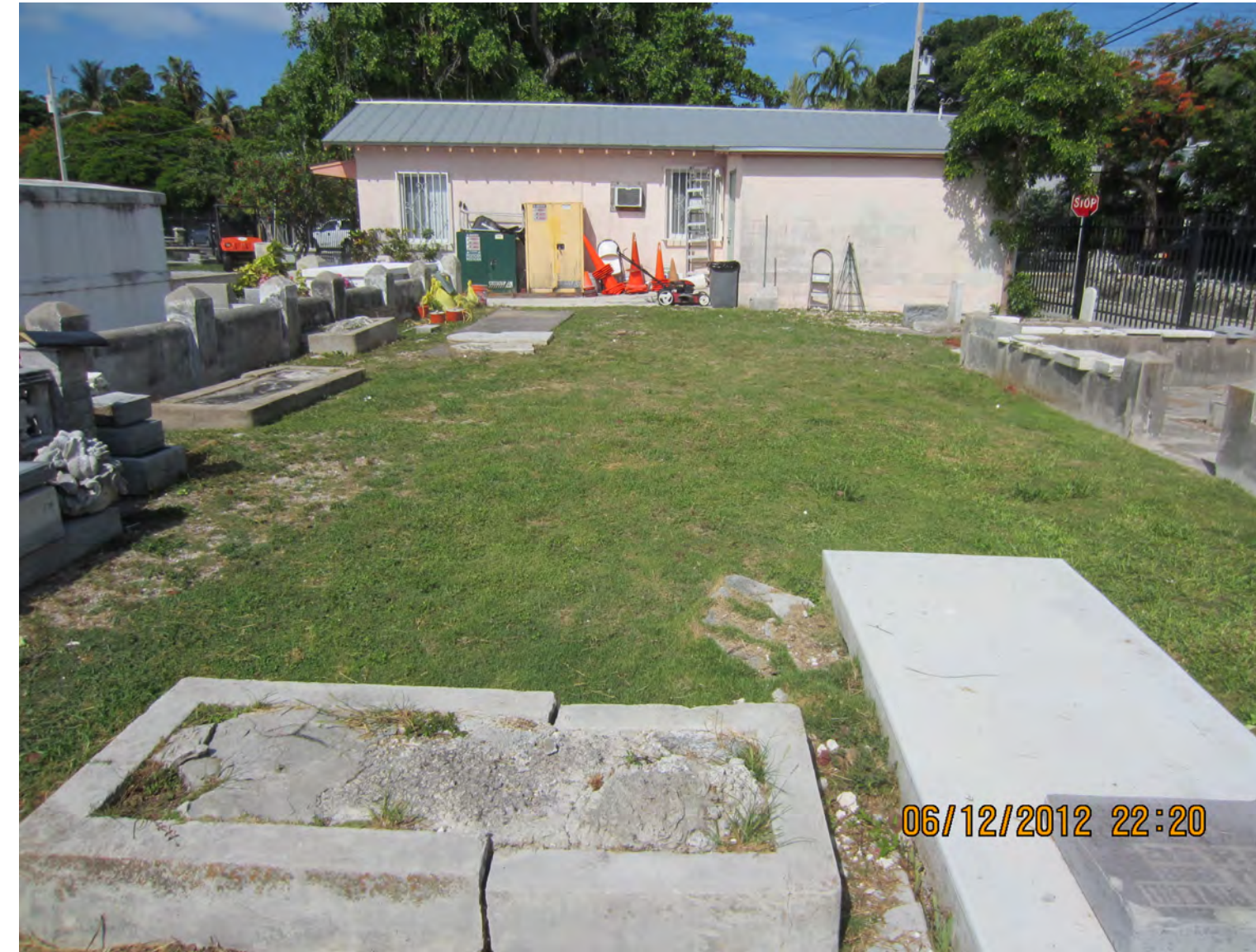
EAST SIDE OF EXISTING SEXTON'S HOUSE
