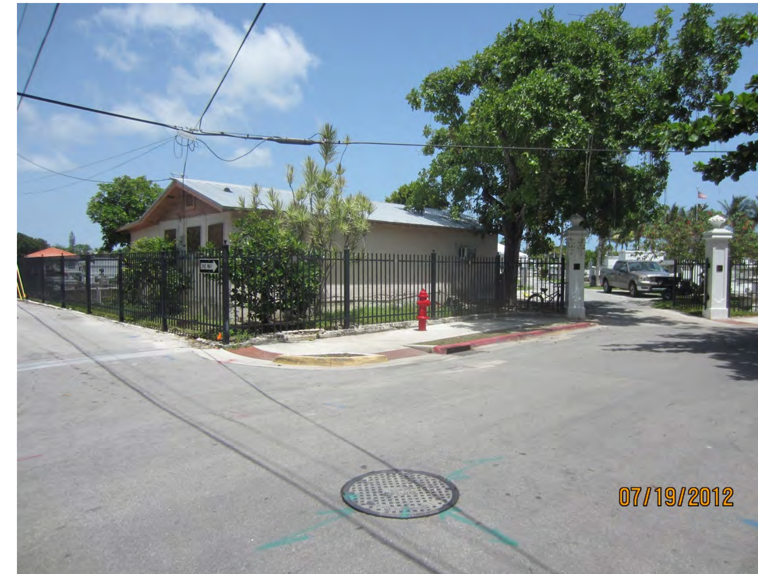
WEST SIDE OF EXISTING SEXTON'S HOUSE AND MAIN ENTRANCE TO THE CEMETARY
