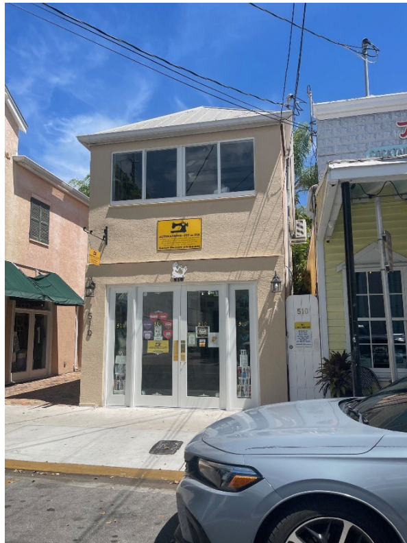
Photo of Property Under Review Front (North) Elevation.
