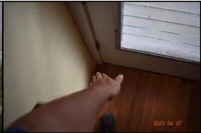
Various sections of flooring were sloped.
