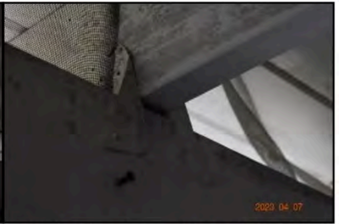
Porch ceiling rafters were properly attached.
