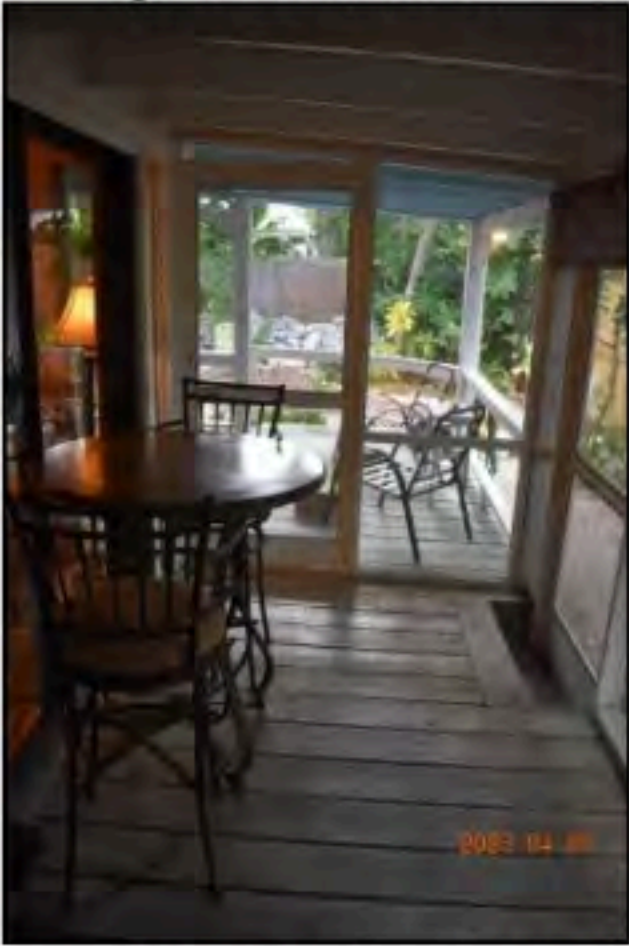
Porch decking was secure but weathered.
