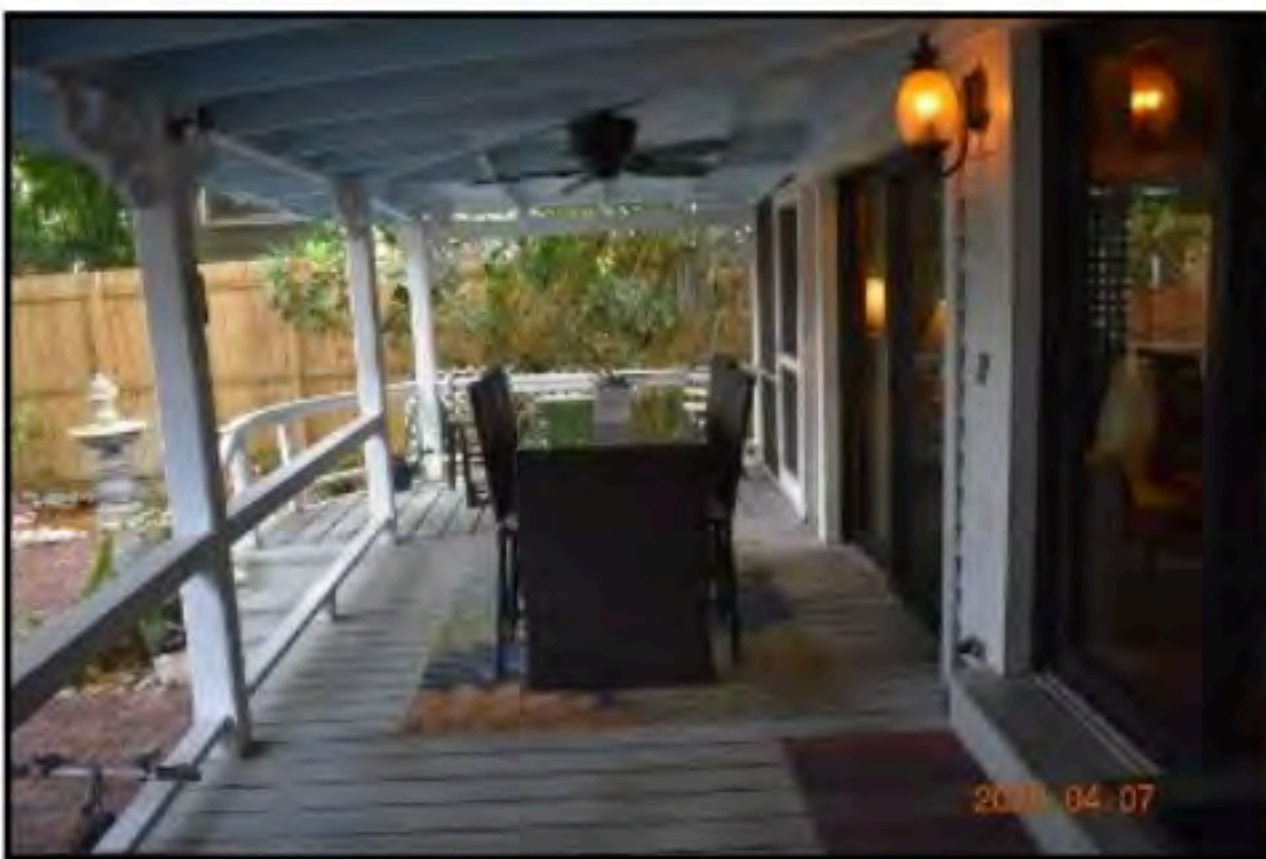
Rear porch posts were secure and in good condition.
