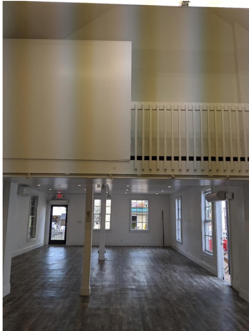
Rear interior showing the first and second levels.
