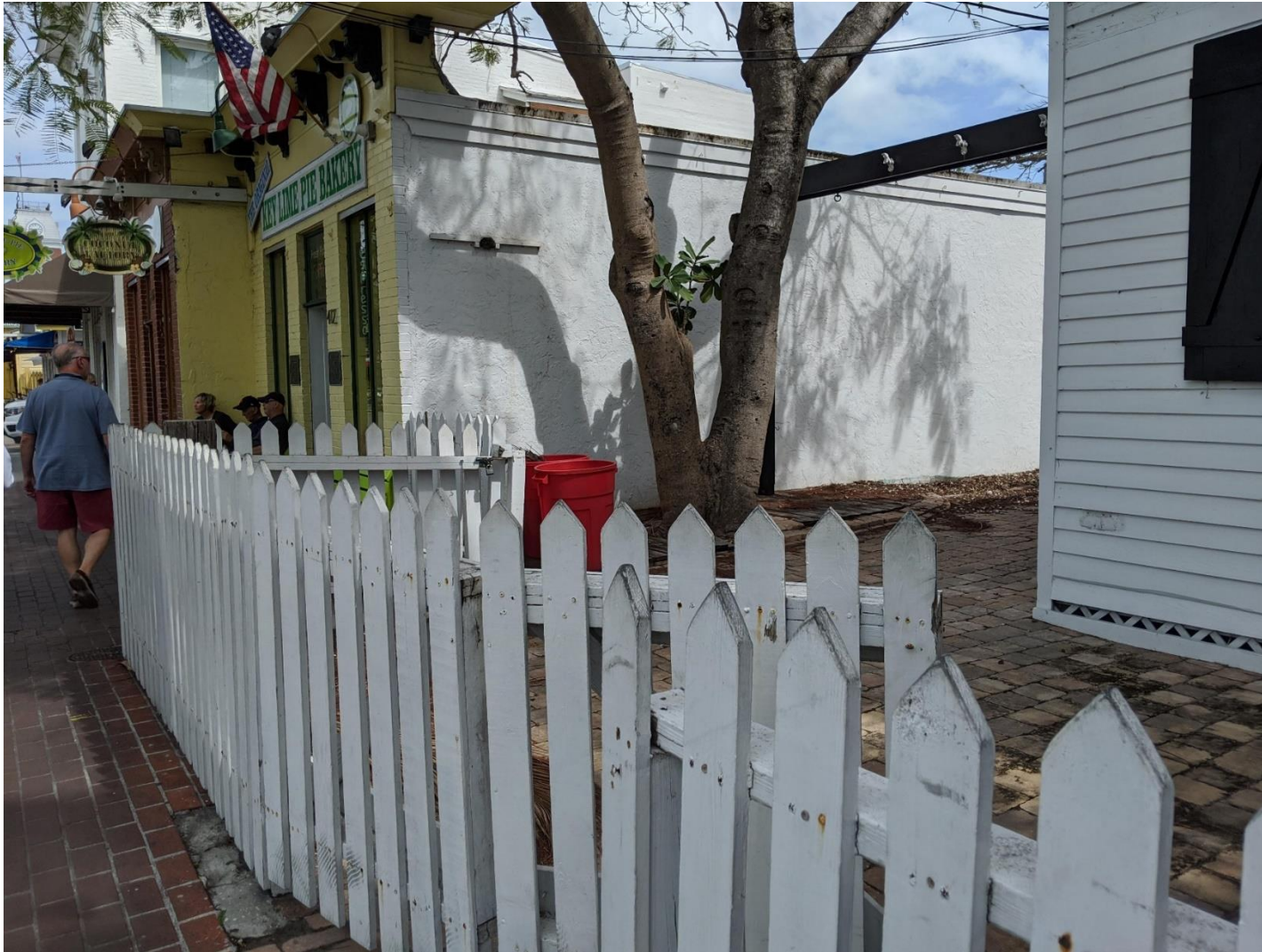
Fence is currently encroaching into the City's right-of-way. Applicant will be either relocating the fence within the property lines or removing the fence all together.
