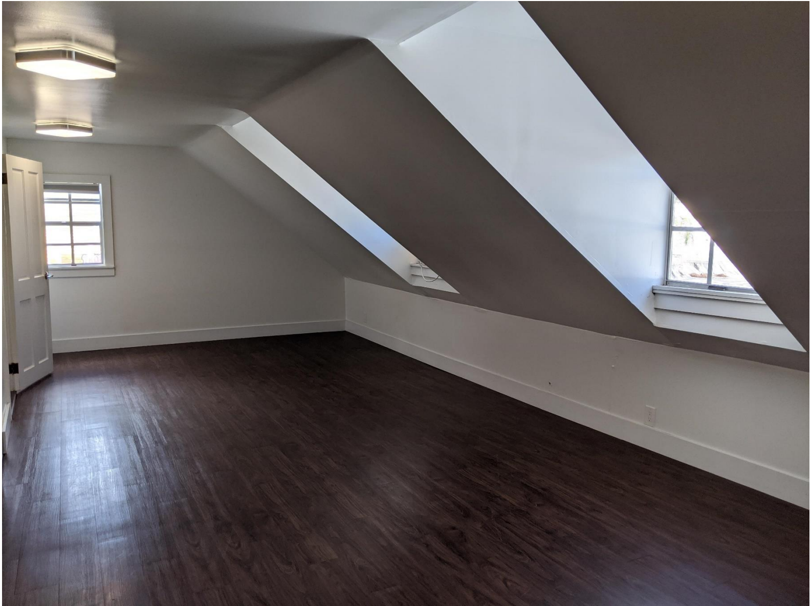
Second floor accessible from an interior staircase will be utilized as a office/ storage space.
