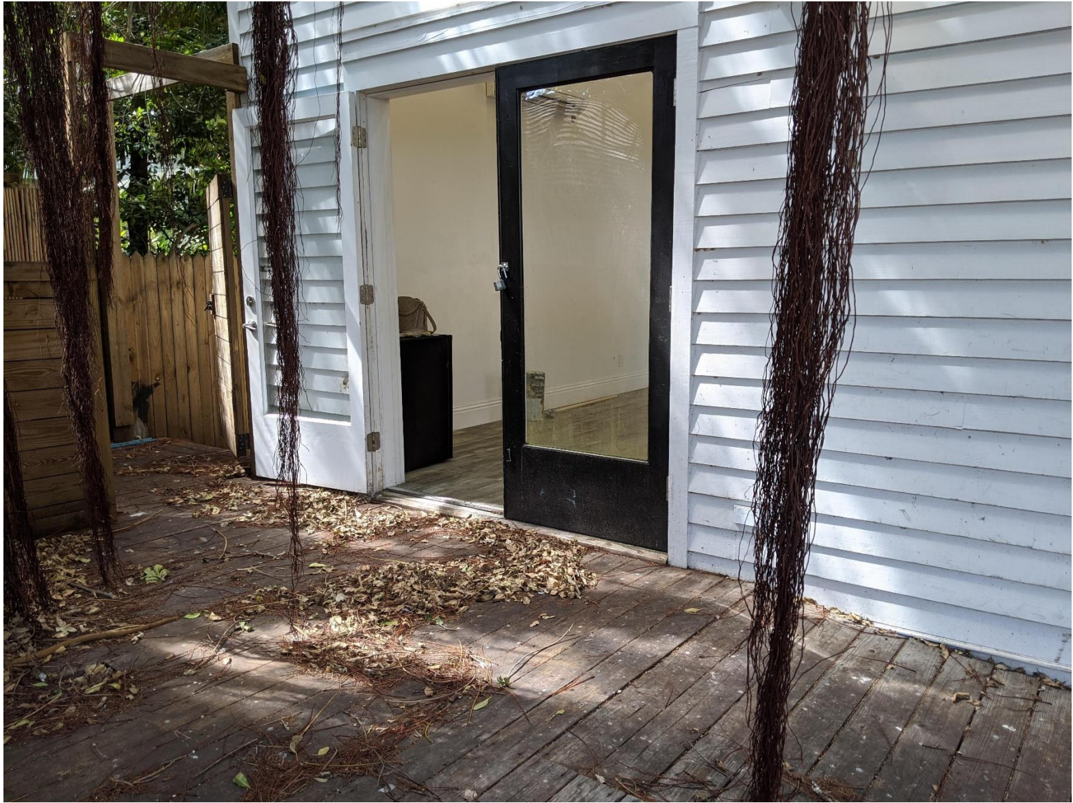
Ground level ADA accessible ramp into the first floor of the structure.
