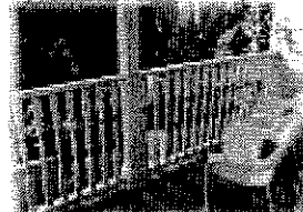
Covered Back Porch Off Master Bedroom
