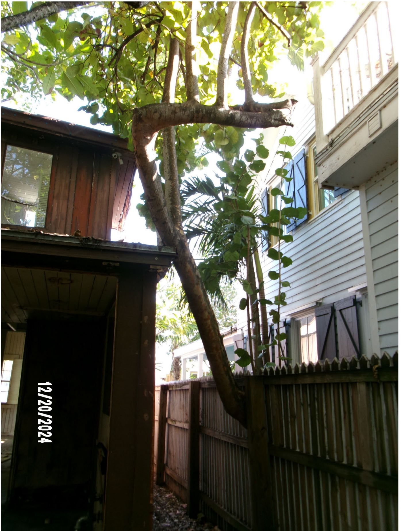
Photo taken from th rear yard of 906 Packer looking at the tree trunk and canopy.
