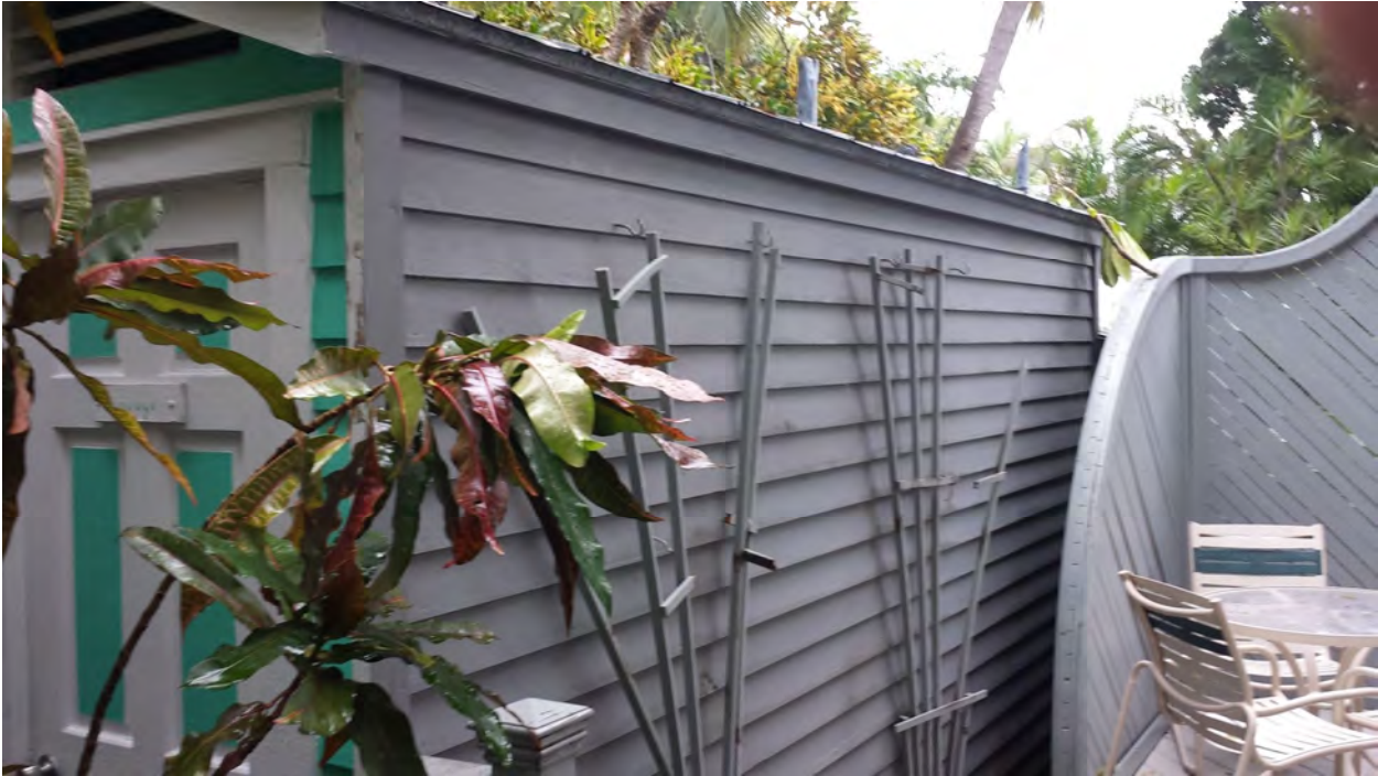
EXISTING STRUCTURE - REAR VIEW
