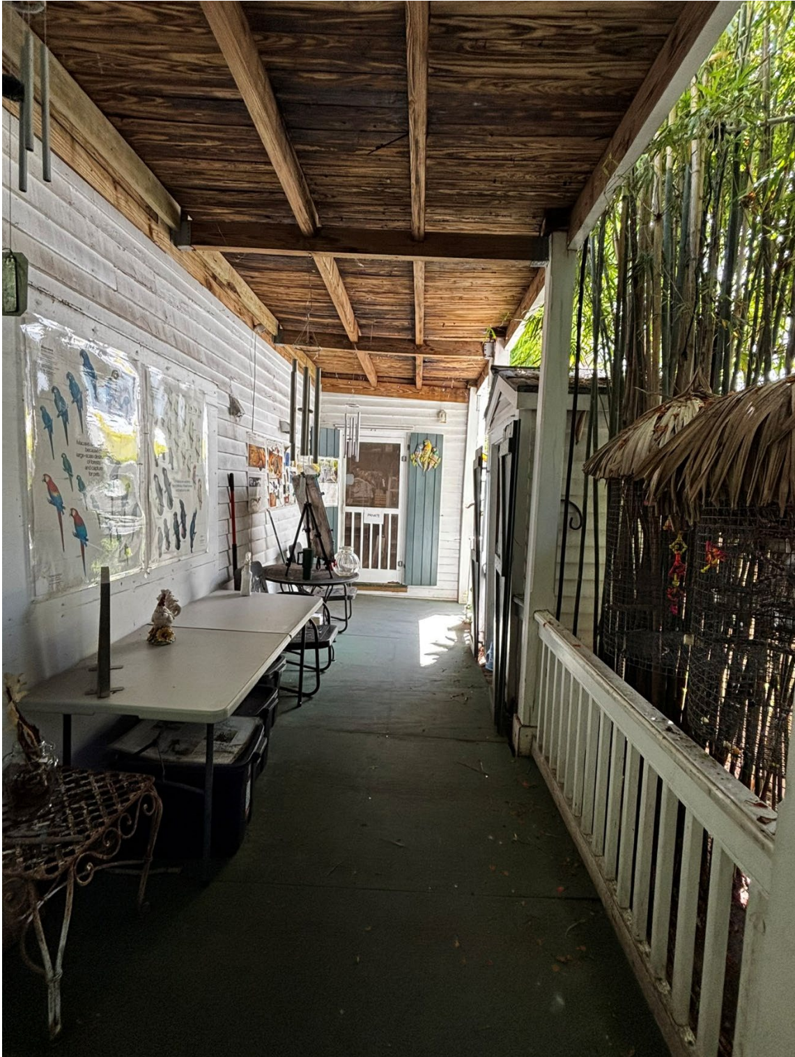
First floor of rear porch of property under review
