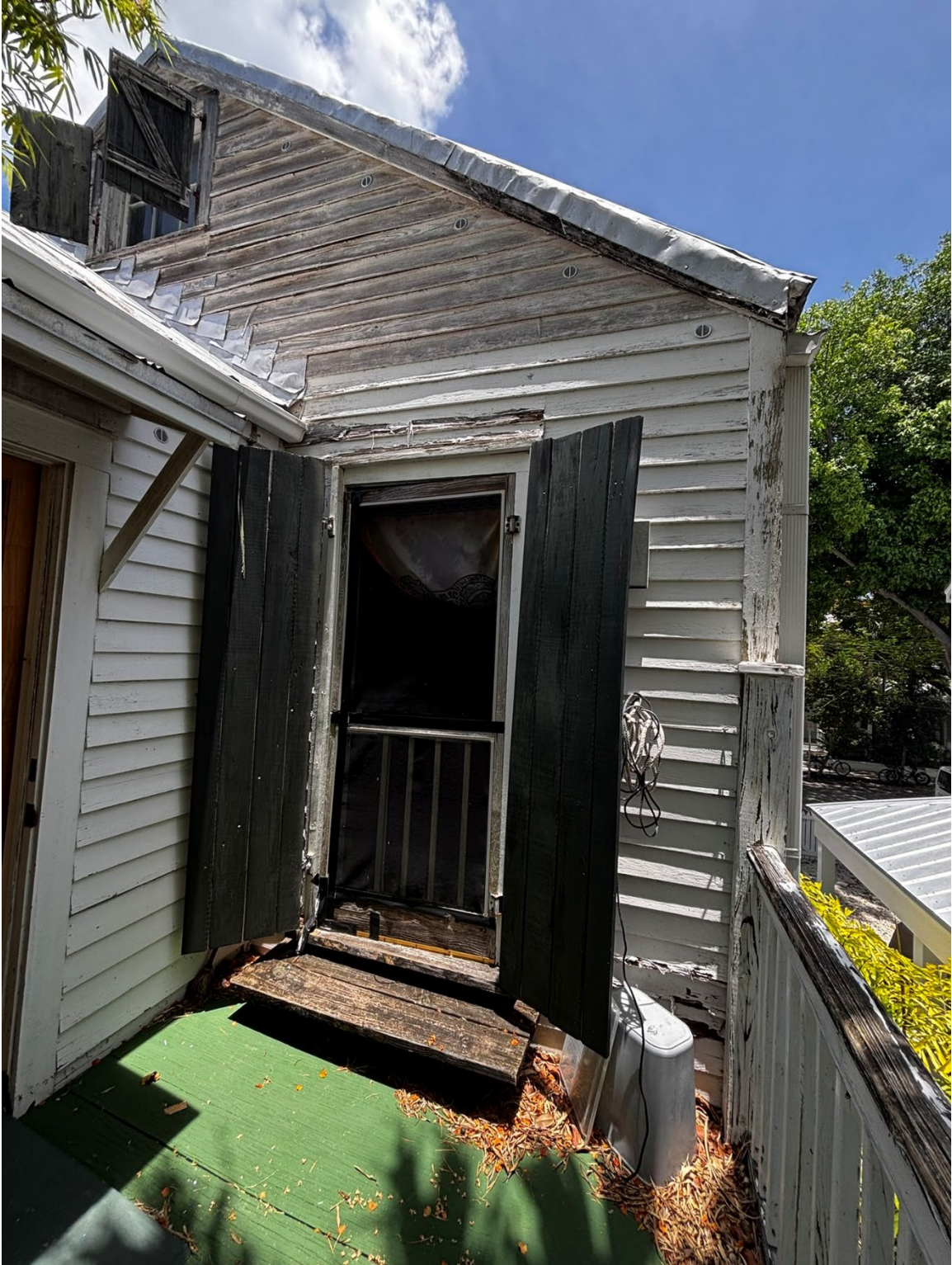
Rear second story porch of property under review.
