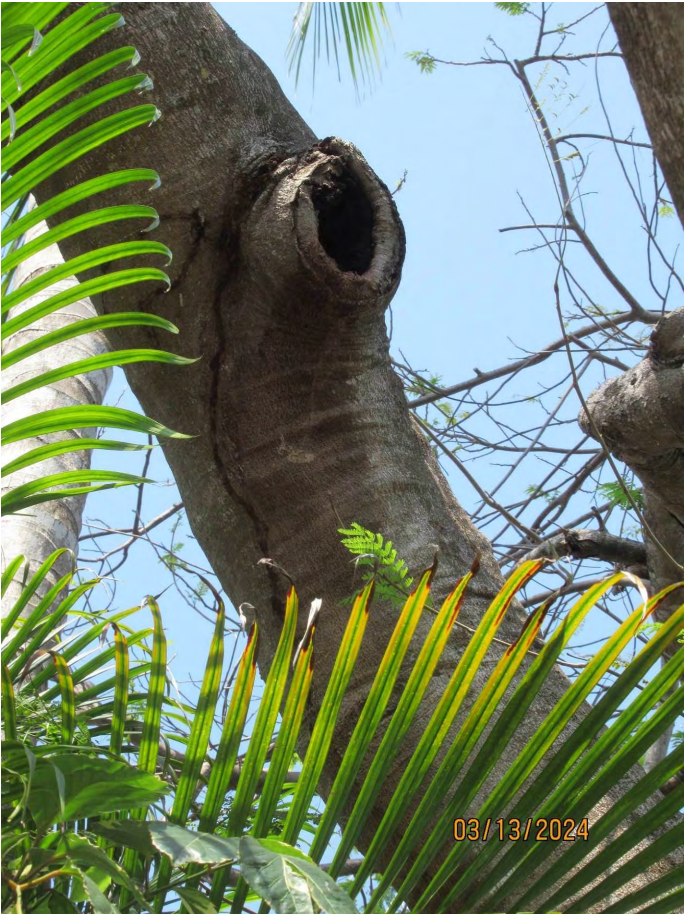
Close up photo of decay area and subterranean termite trail, view 1.
