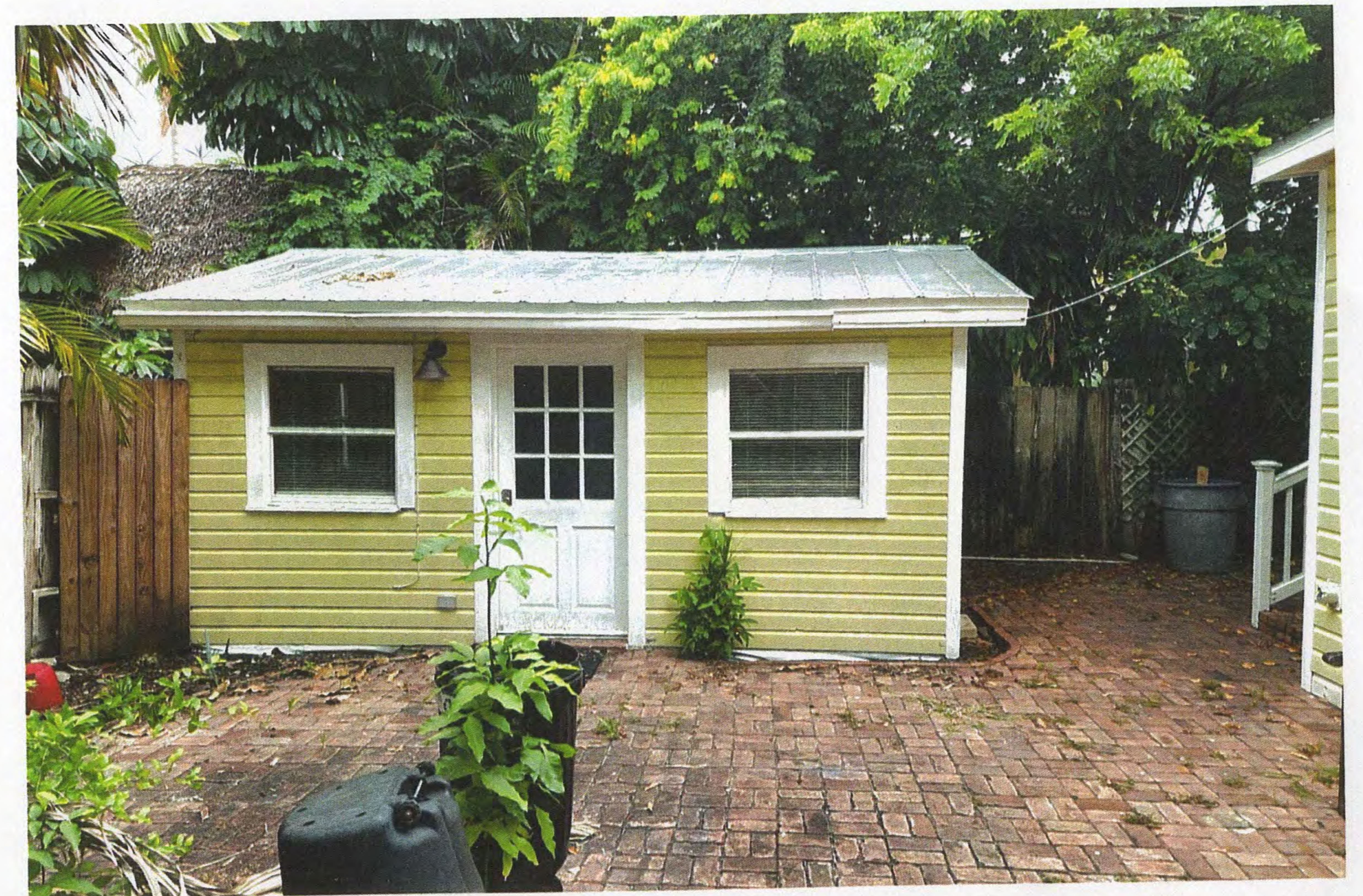
Shed built in set-back area to be removed
