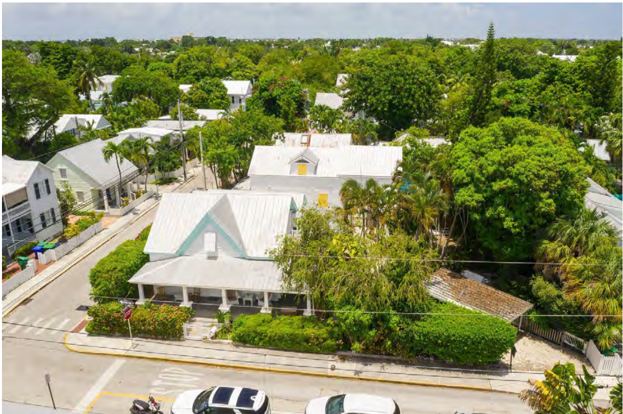
Aerial photograph of the site under review.
