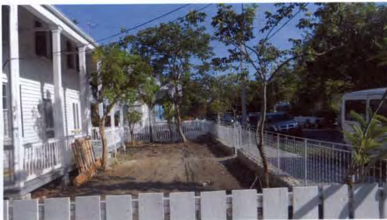
View of front yard. Existing fencing to remain. New pavers from house to sidewalk.
