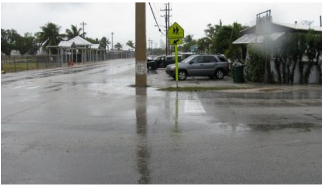
Typical drainage pattern at intersection
