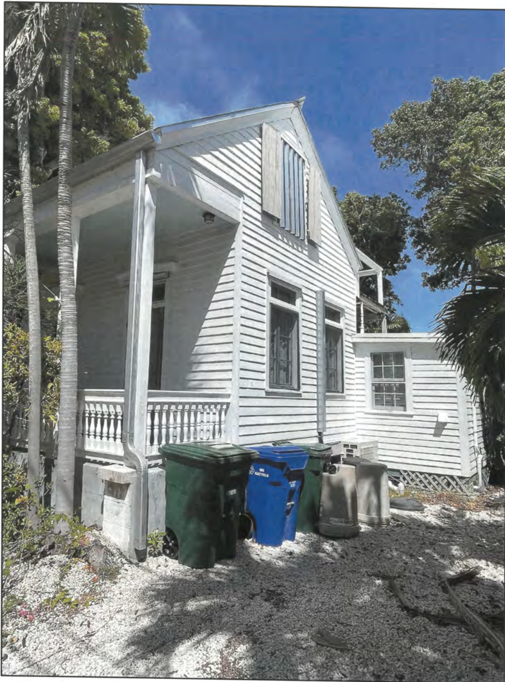
VIEW FROM SIDE OF THE HOUSE (EXISTING SOUTH ELEVATION)
