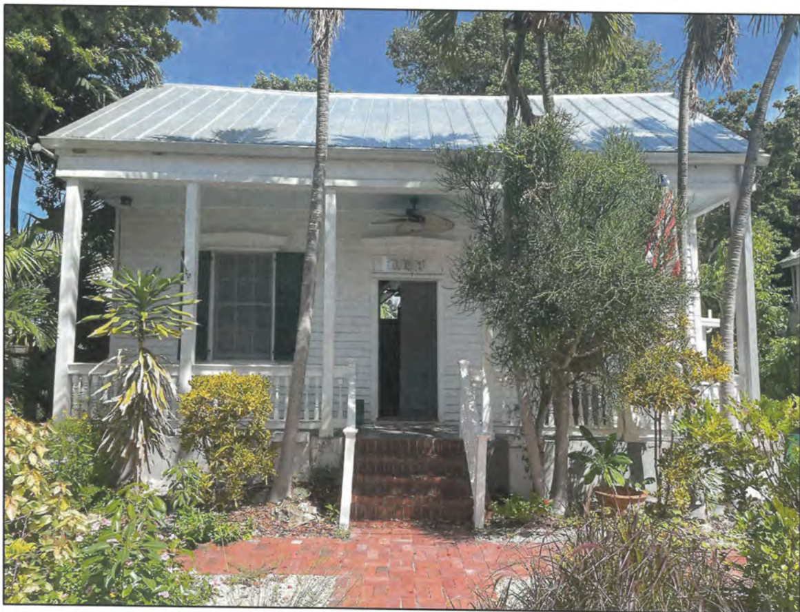
VIEW FROM CATHOLIC LANE (EXISTING WEST ELEVATION)
