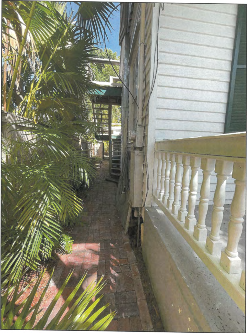
VIEW FROM SIDE OF THE HOUSE (EXISTING NORTH ELEVATION)
