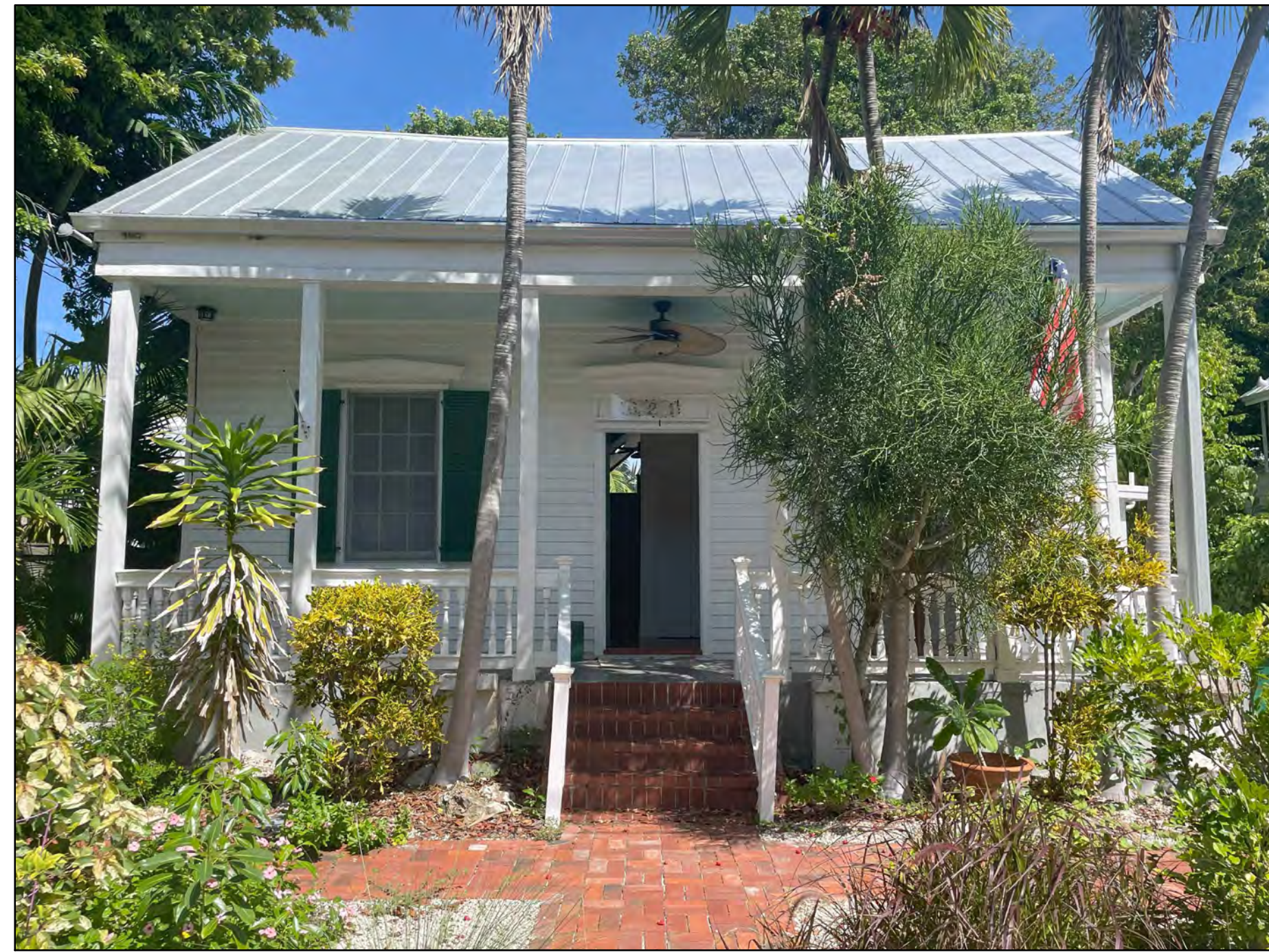
4 A8 VIEW OF THE FRONT OF THE HOUSE (EXISTING WEST ELEVATION) SCALE: N.T.S.
