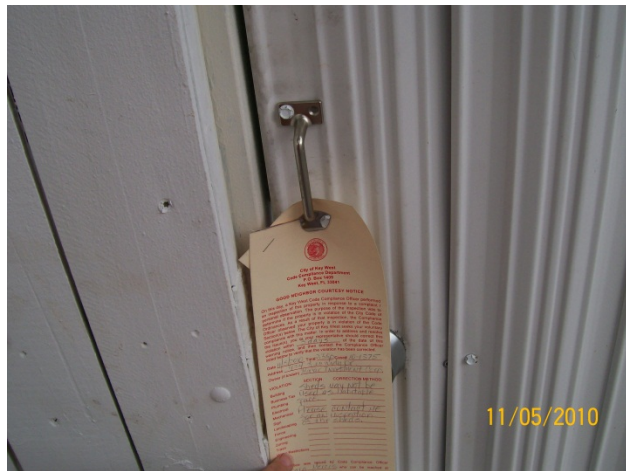
Photo #3, door hanger attached to locked gate
