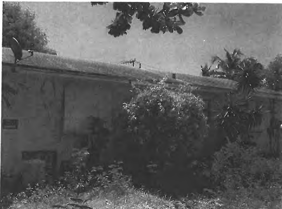
Rear View & Electrical Panel 8/21/12
