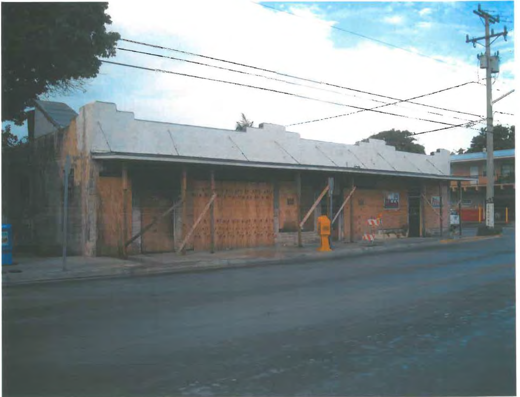
Building after 2008 fire.
