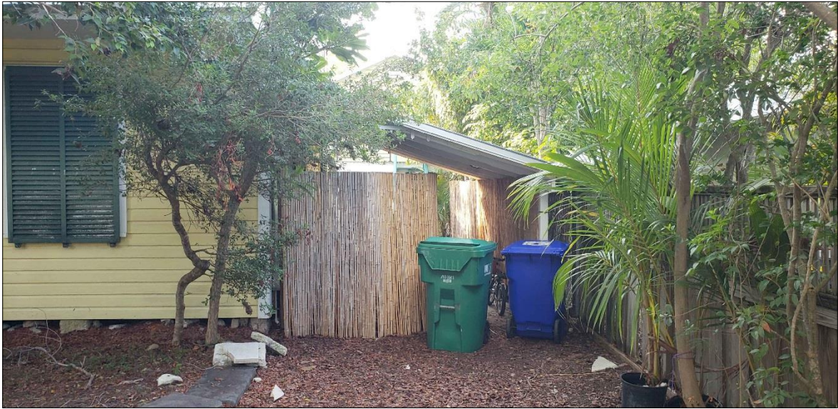
1226 South St, Carport – Front
