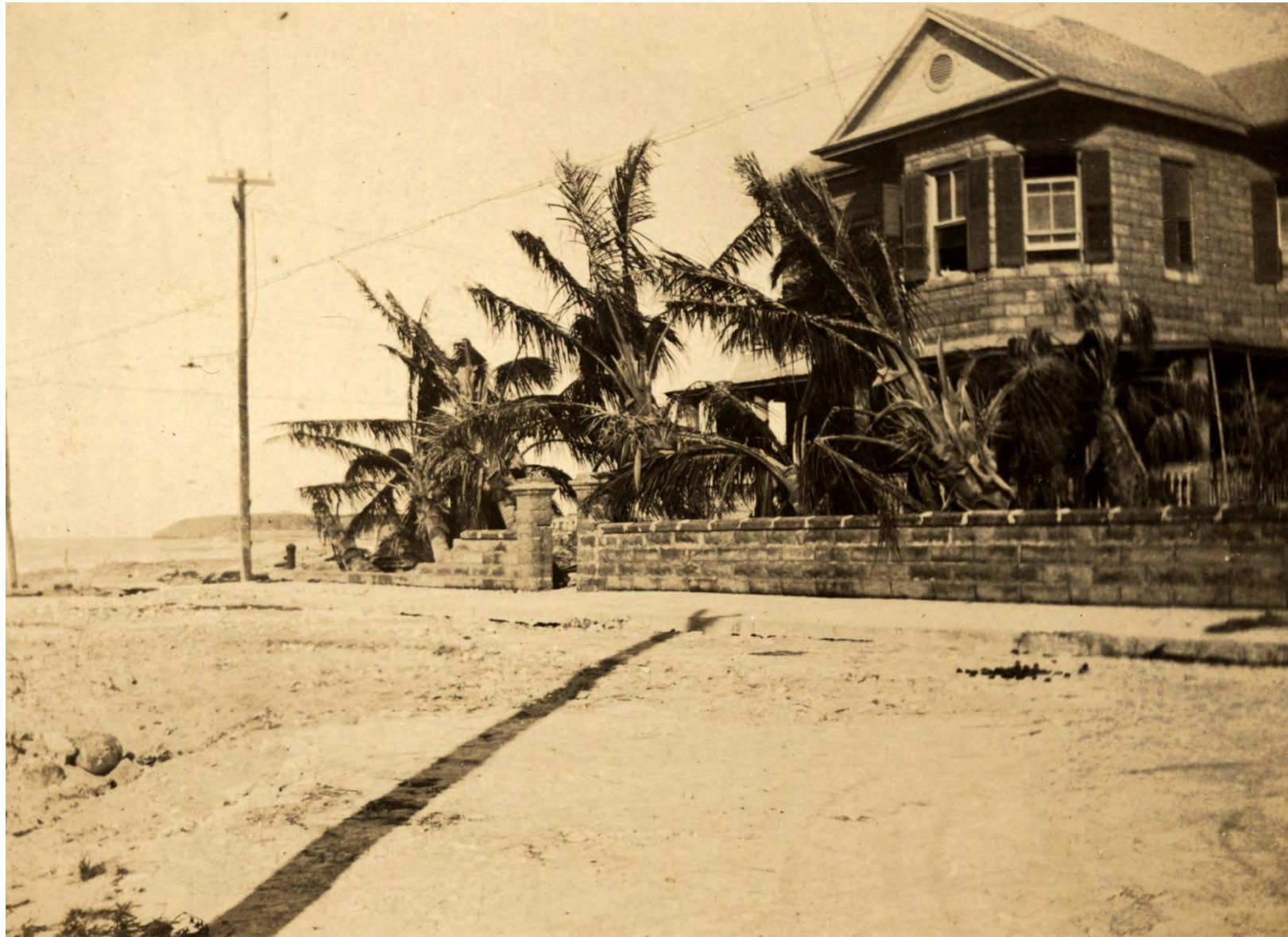
401 South Street in 1919 after hurricane. Monroe County Library.
