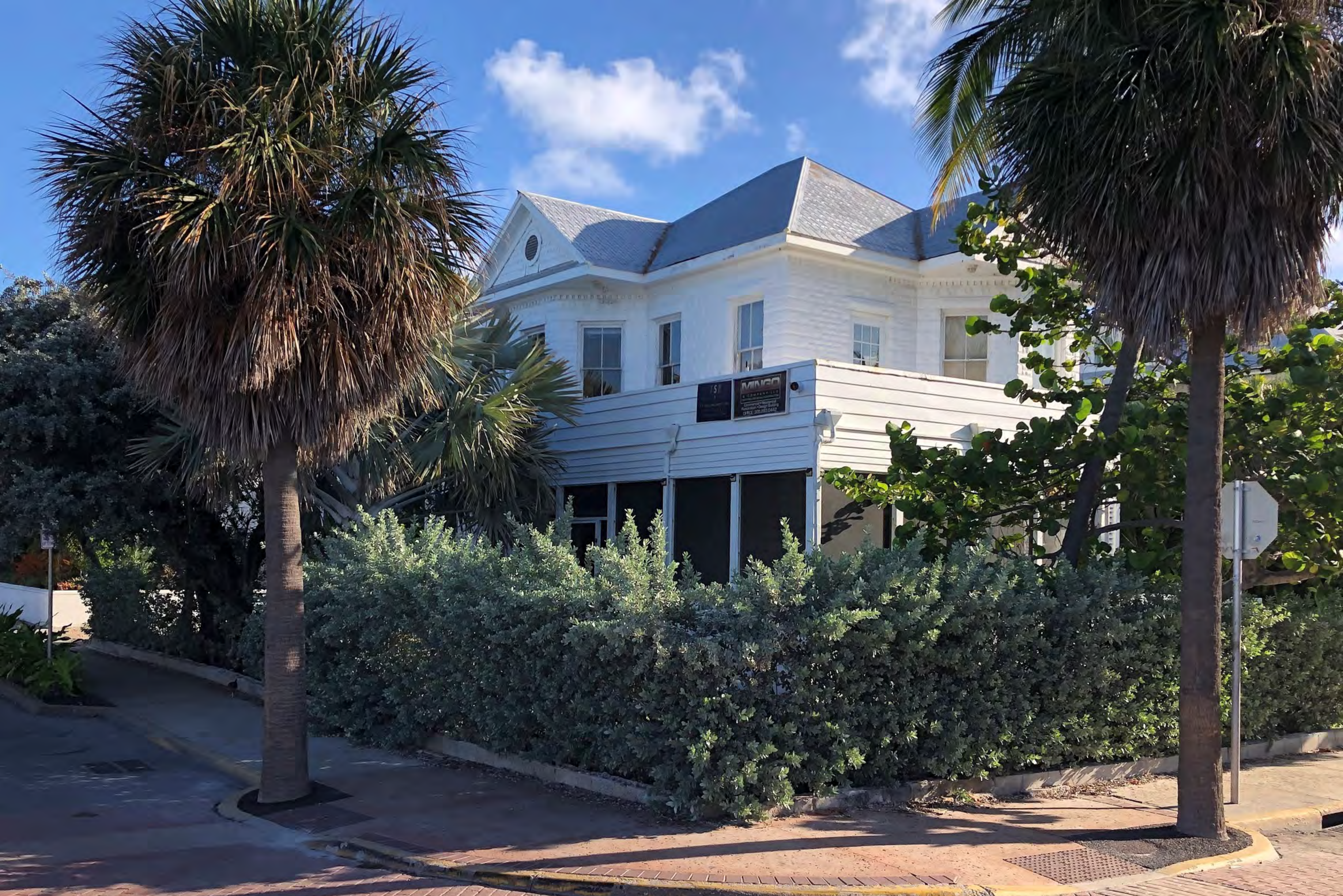
401 SOUTH STREET: SOUTHERN MOST CORNER, SOUTH STREET / WHITEHEAD ELEVATION
