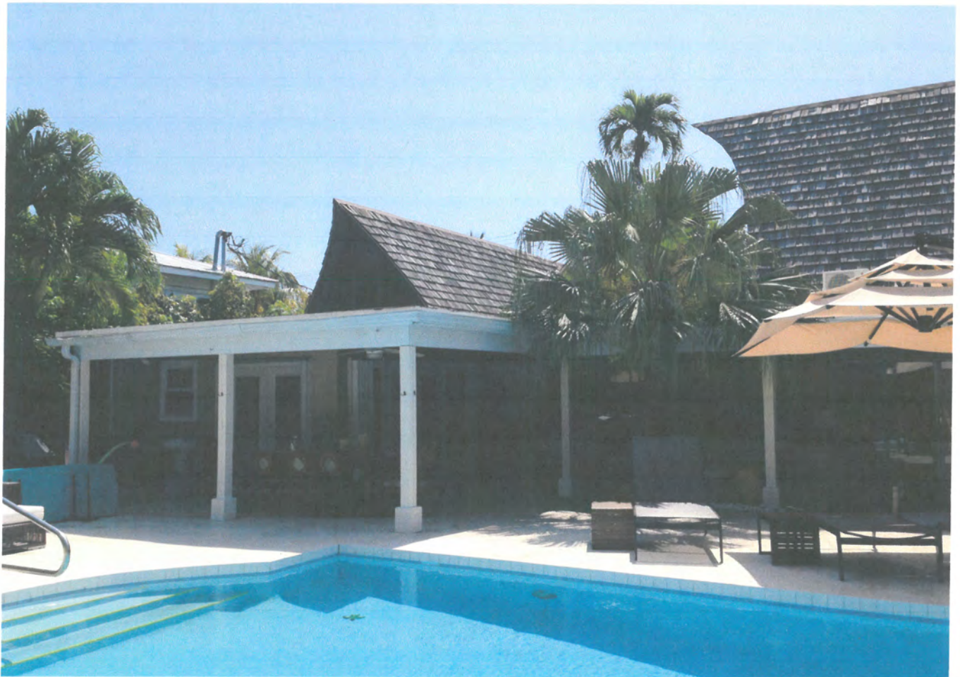
1415 ALBERTA - VIEW LOOKING SOUTHWEST FROM POOL DECK
