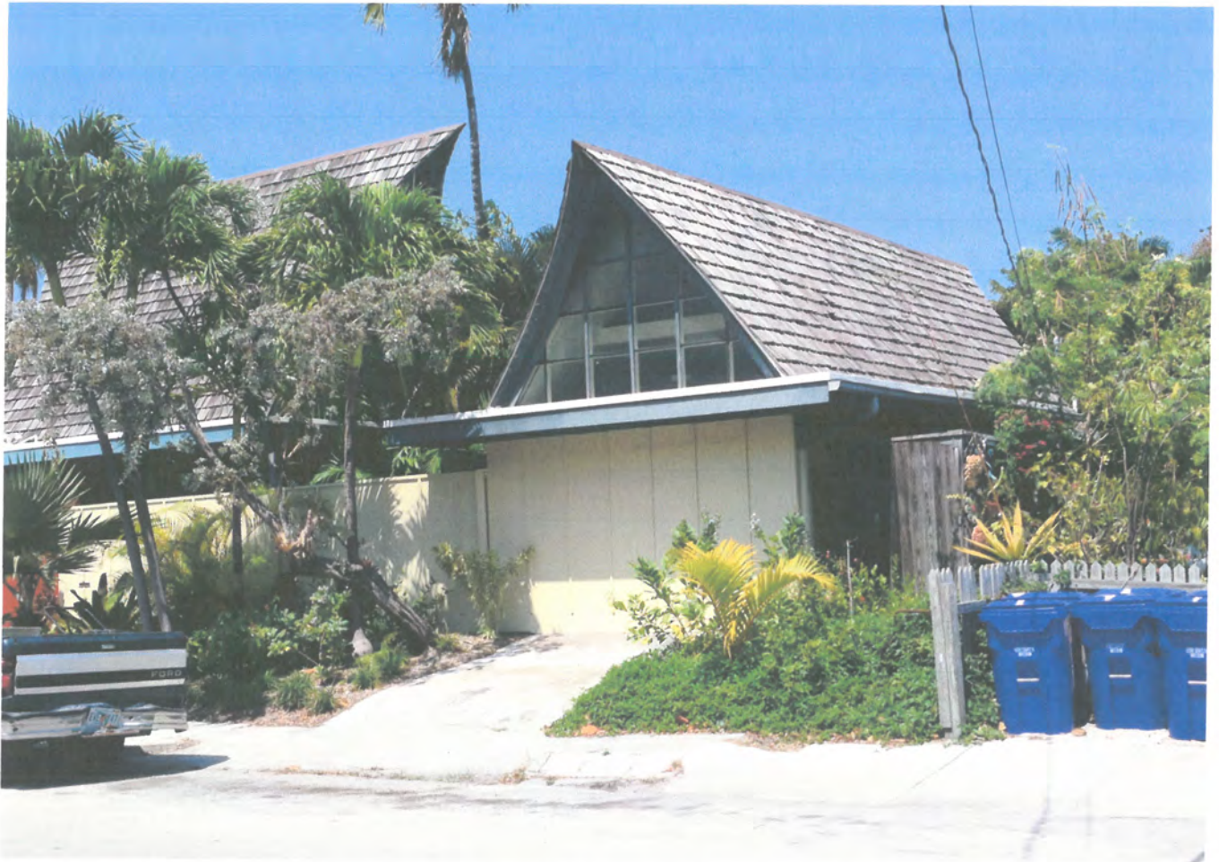
1415 ALBERTA VIEW FROM SOUTHWEST
