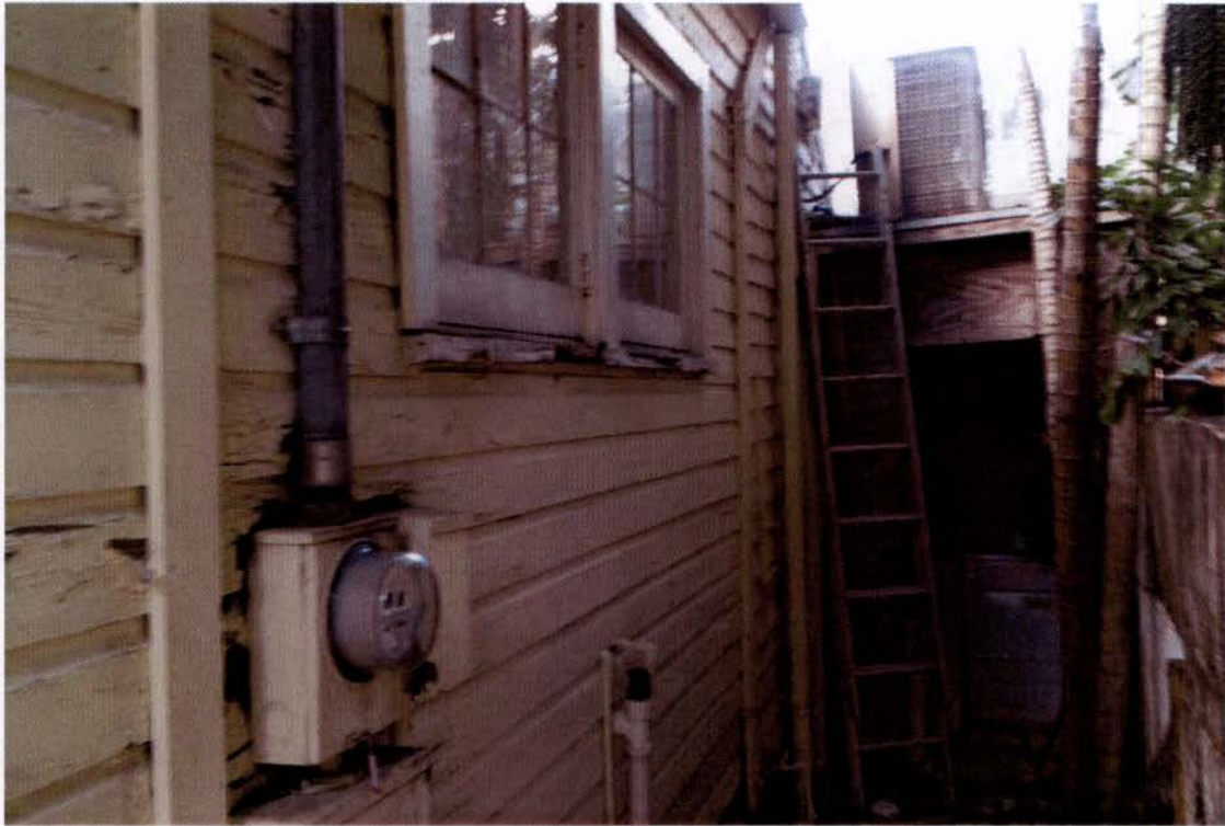
SHED AT REAR ON SOUTHEAST SIDE OF EXISTING STRUCTURE
