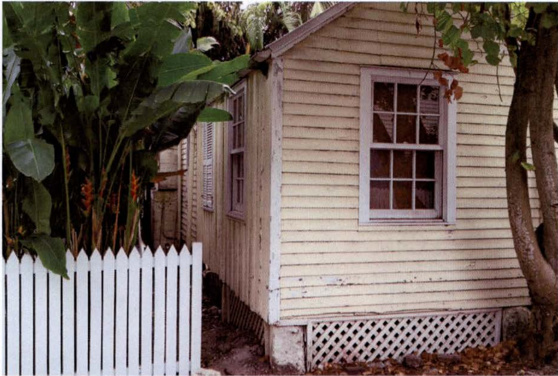
NORTHEAST ELEVATION TOWARD REAR OF EXISTING STRUCTURE
