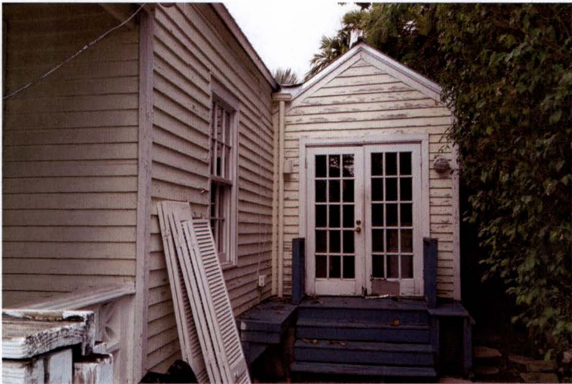
DECK ON SOUTHEAST SIDE OF EXISTING STRUCTURE
