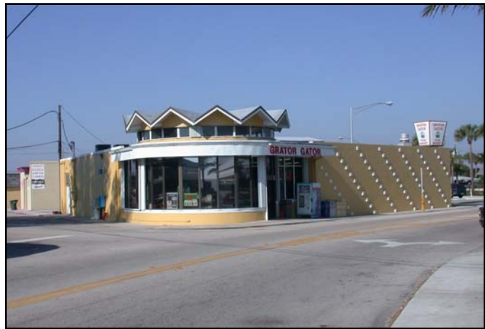
A mid-twentieth century, commercial building with a folded-plate roof.
