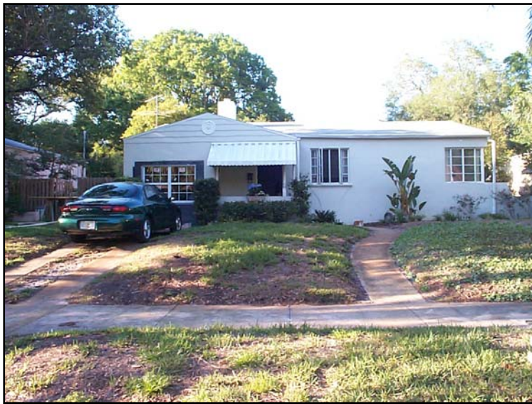
Renovated vernacular home within the Harborview Neighborhood, Tampa, Florida.
