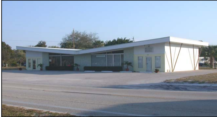
Constructed as a boat dealership, this 1955 building has an elevated “winged” roof to accommodate boat masts.
