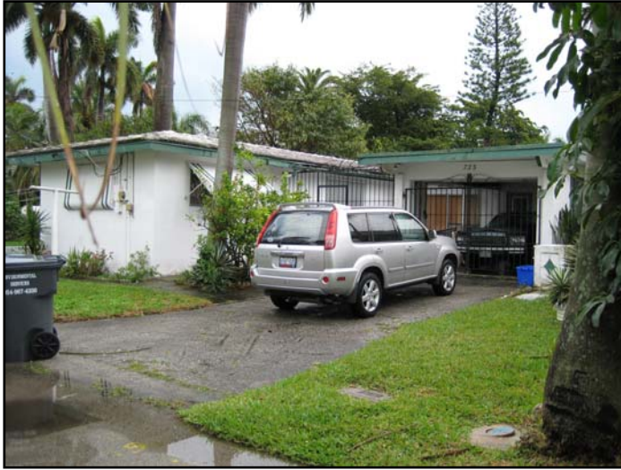
A typical 1959, masonry house on Hollywood Boulevard, Broward County, Florida.
