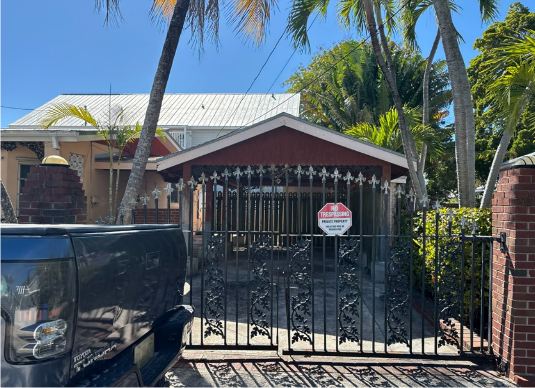
1012 Howe Street Carport and Front gate
