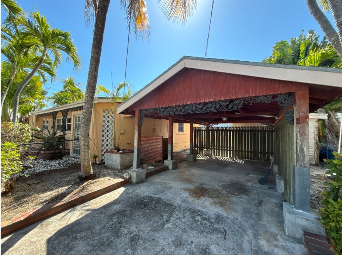
1012 Howe Street Carport
