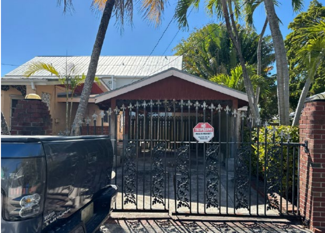
Photo of Property Under Review Showing Front Gate and Carport.
