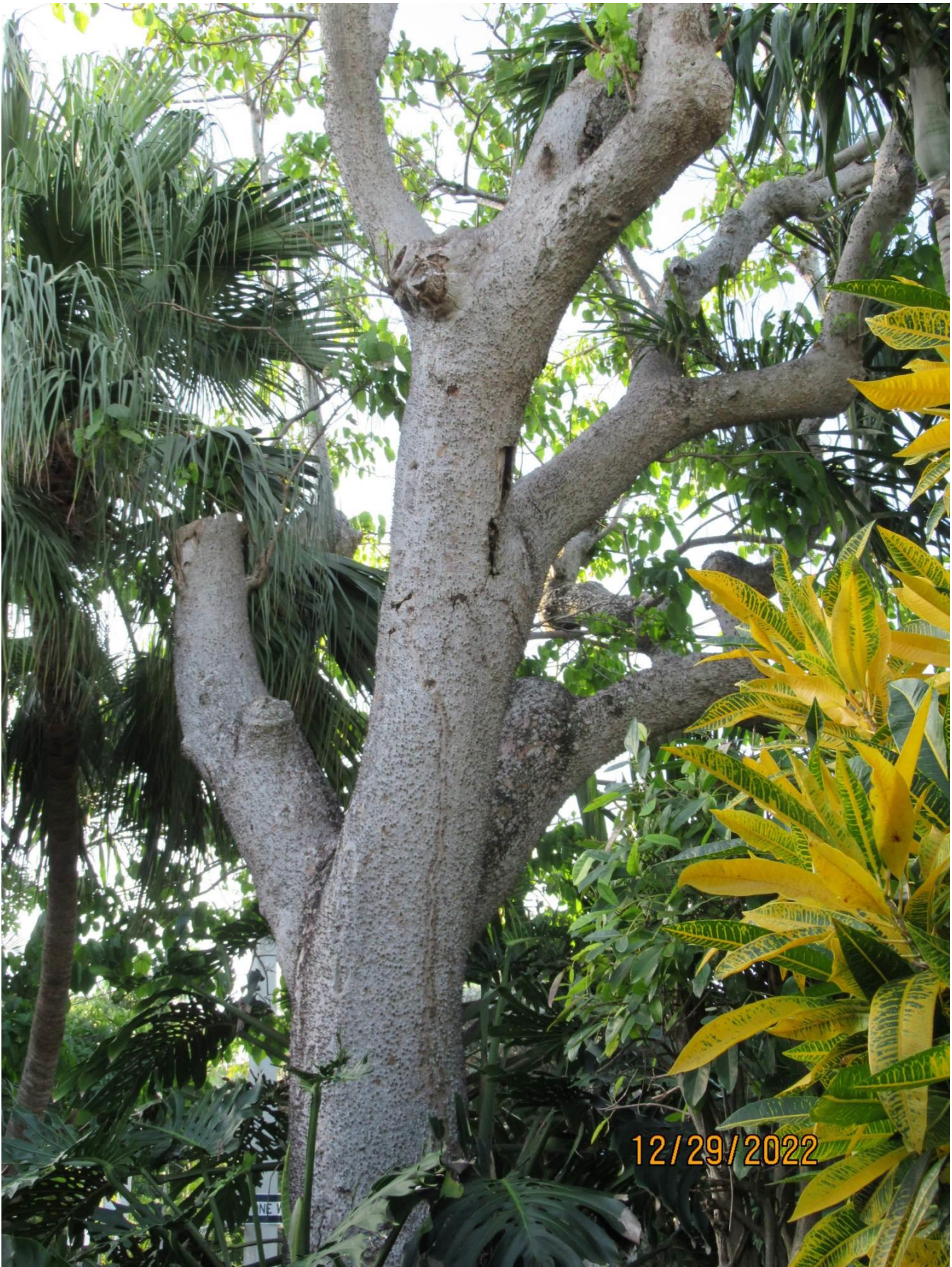
Photo of main canopy branches showing decay, view 4.
