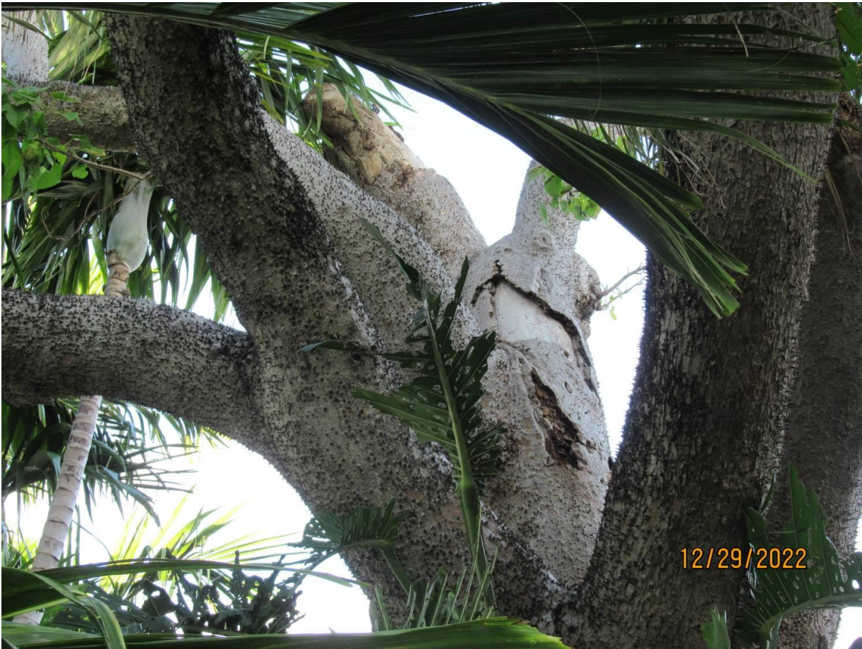
Closeup photo of main canopy branches showing decay, view 3.
