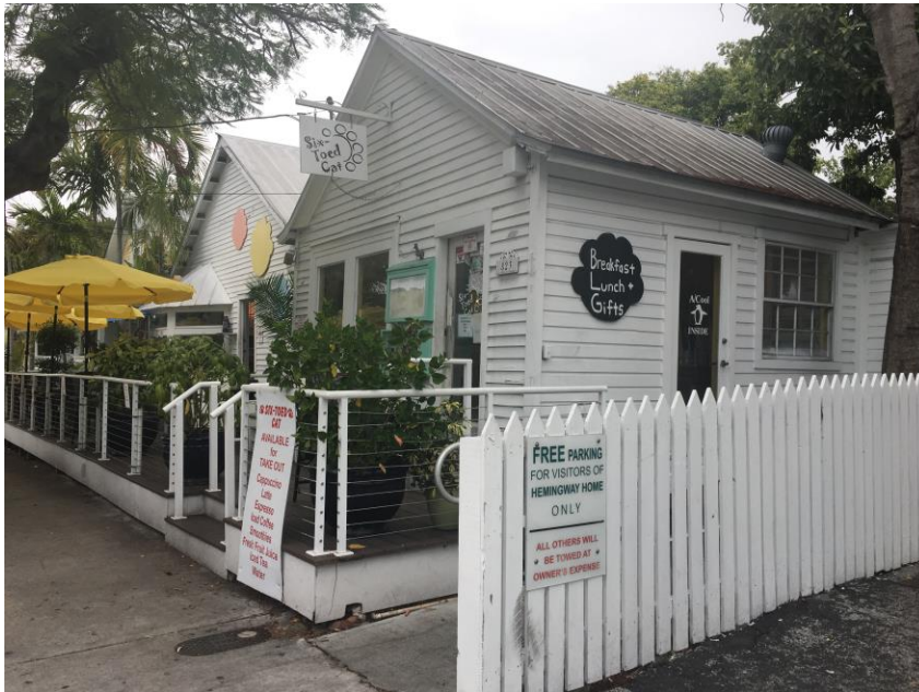
The Six-Toed Cat Café' existing non-conforming retail area.
