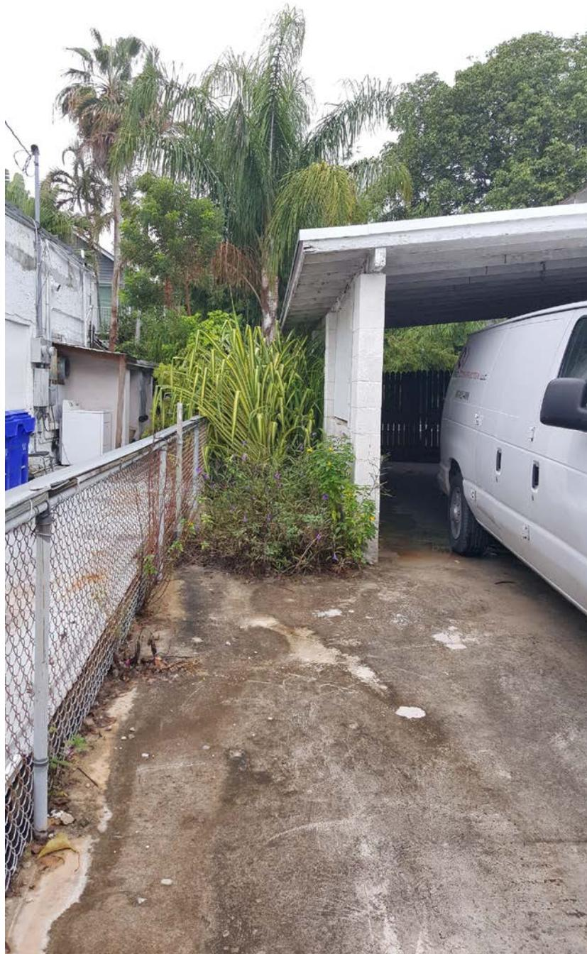
1212 Margaret Street – View of carport illustrating simple construction and concrete block supporting wall
