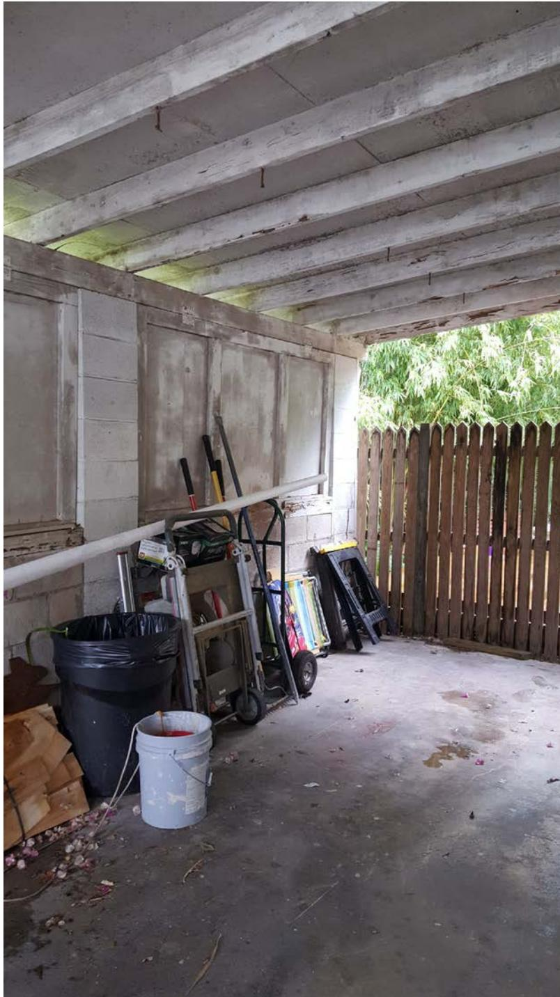
1212 Margaret Street – View of carport illustrating simple construction and concrete block supporting wall
