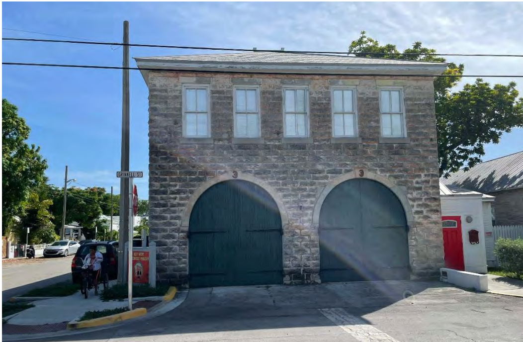
1024 Grinnell Street – opposite corner to subject site (northwest).
