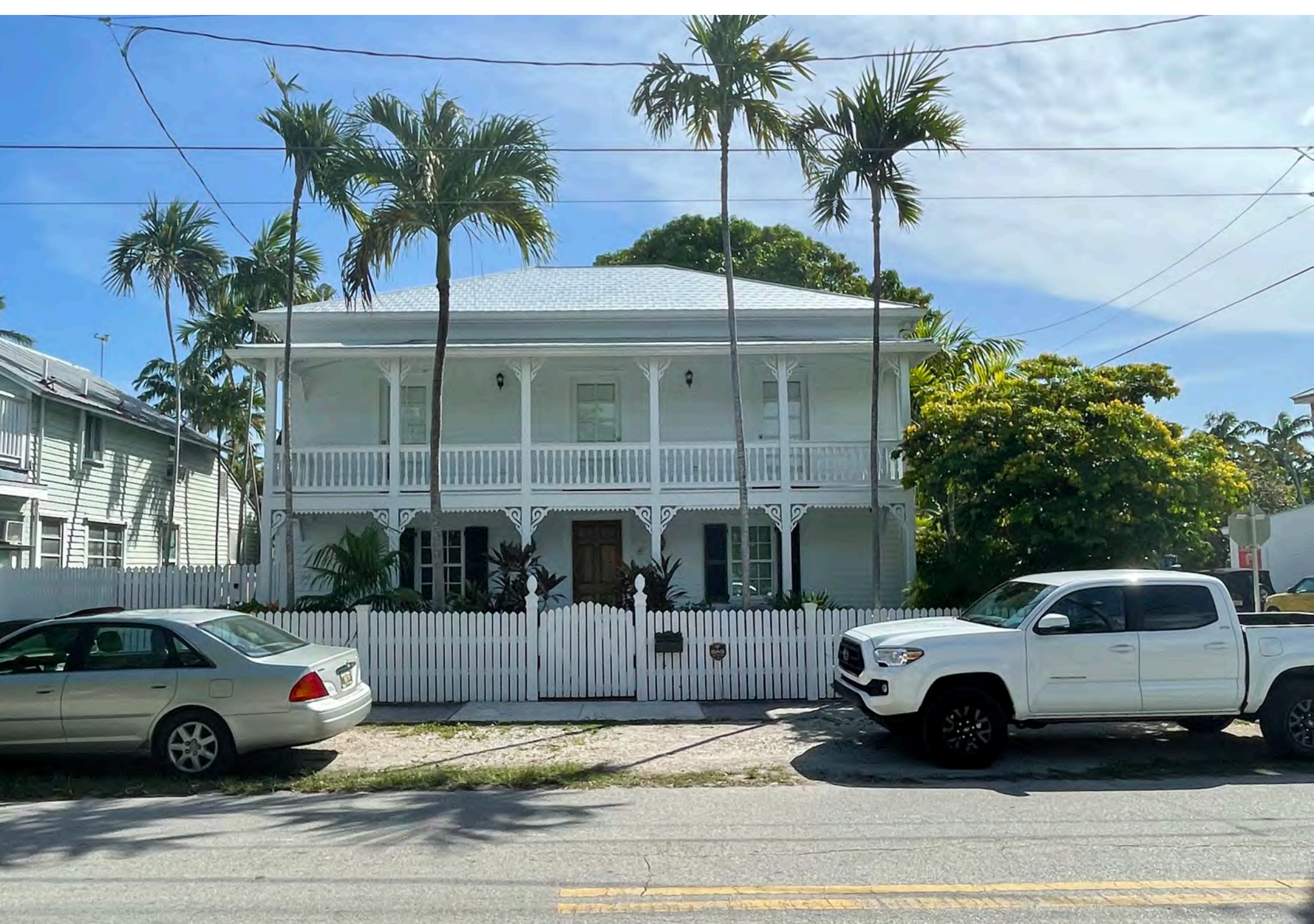
1100 GRINNELL STREET: NORTHEAST (STREET VIEW)
