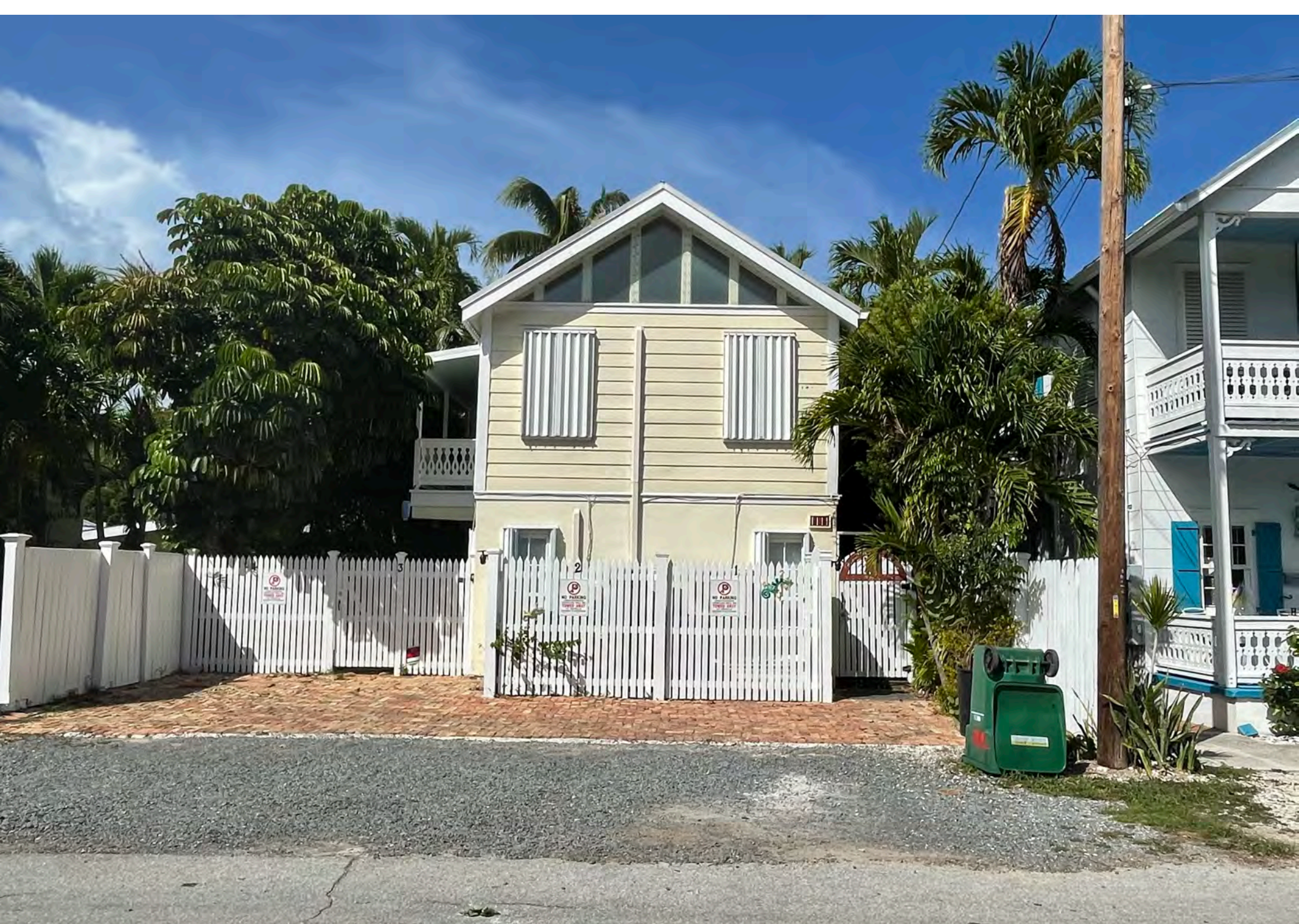
1111 GRINNELL STREET: SOUTHWEST (STREET VIEW)
