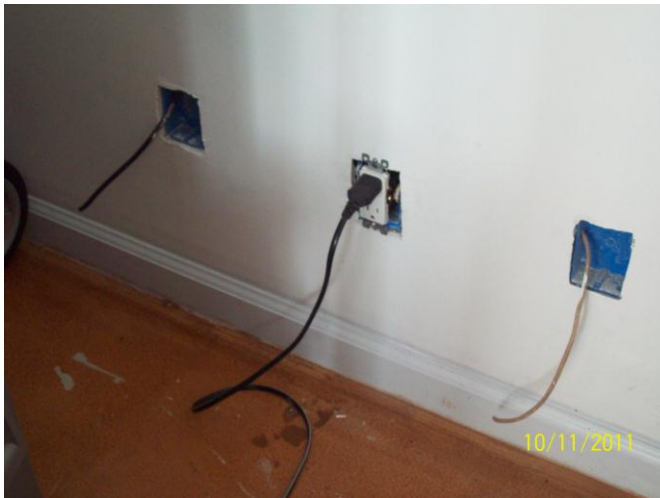
Electrical wiring installed in kitchen, bedroom, and outside flood lights without permits, by Vincent, an unlicensed contractor.
