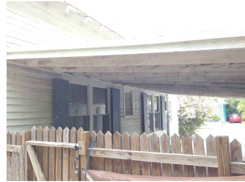
FIGURE 3 WINDOW TO BE SAVED & SECOND WINDOW EXPOSED
