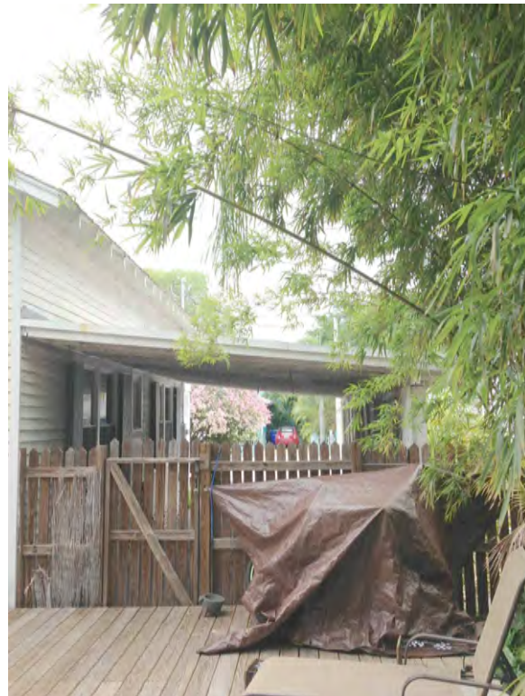
FIGURE 4 REAR VIEW OF CAR PORT
