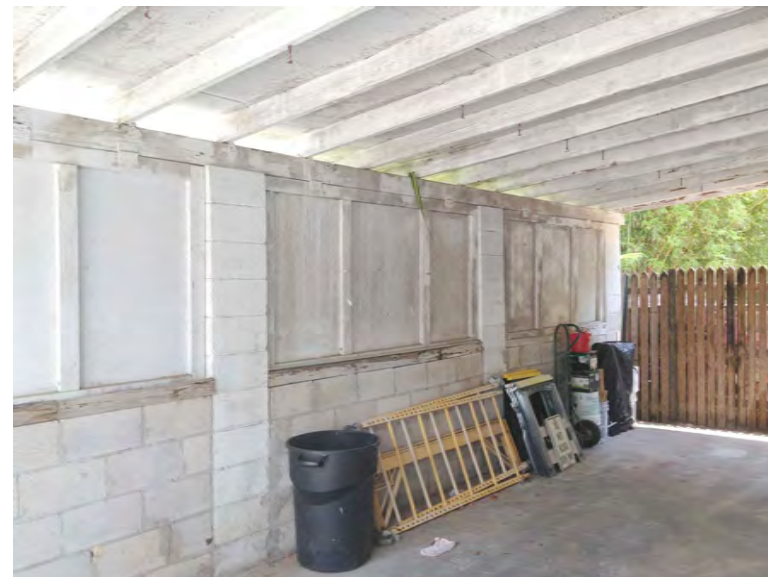
FIGURE 5 INTERIOR VIEW OF CAR PORT
