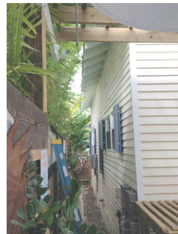
FIGURE 6 REAR RIGHT VIEW OF HOUSE
