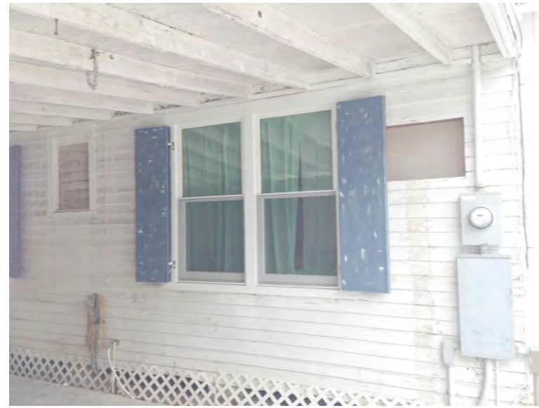
FIGURE 2 WINDOW TO BE EXPOSED
