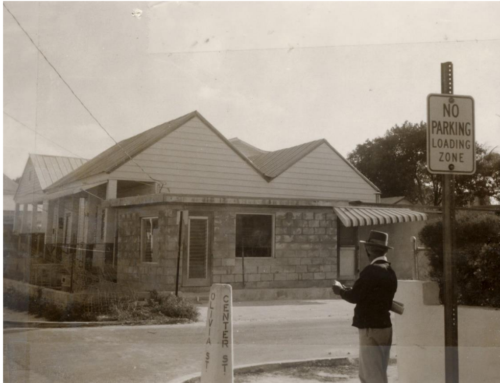
Portions of the corner cmu building are still standing. The one-story structure with two sawtooths was demolished. Photograph circa 1965 from the Monroe County Library.
