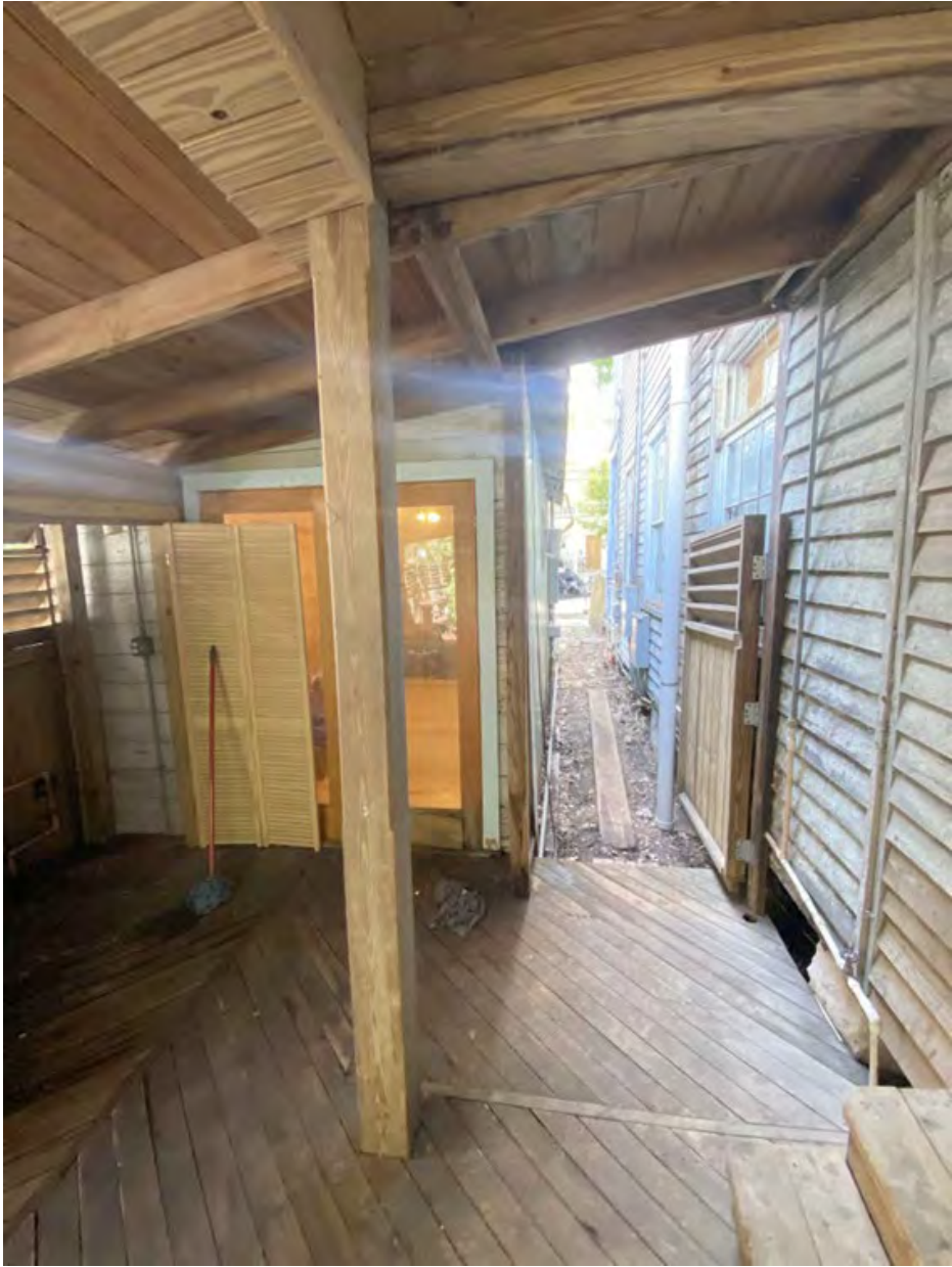
Shed roof, carport / storage structure view.
