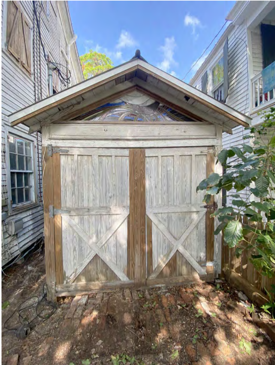
Carport / storage structure view.
