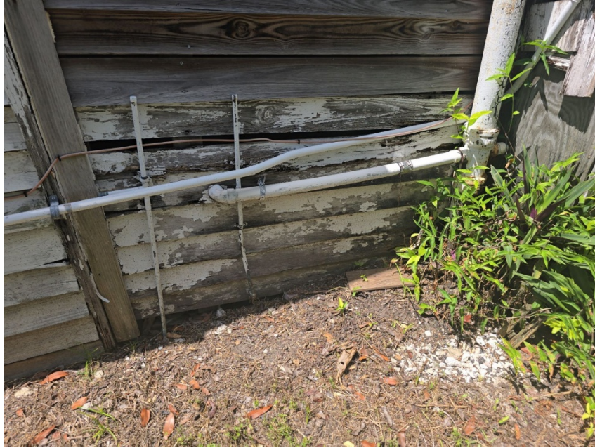
CONDITION OF EXTERIOR SIDING
