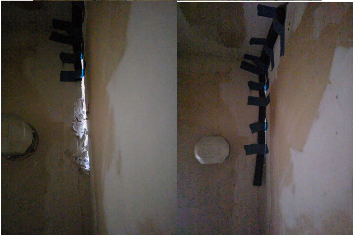
DETERIORATED WALL CONDITION (SEPARATION)
