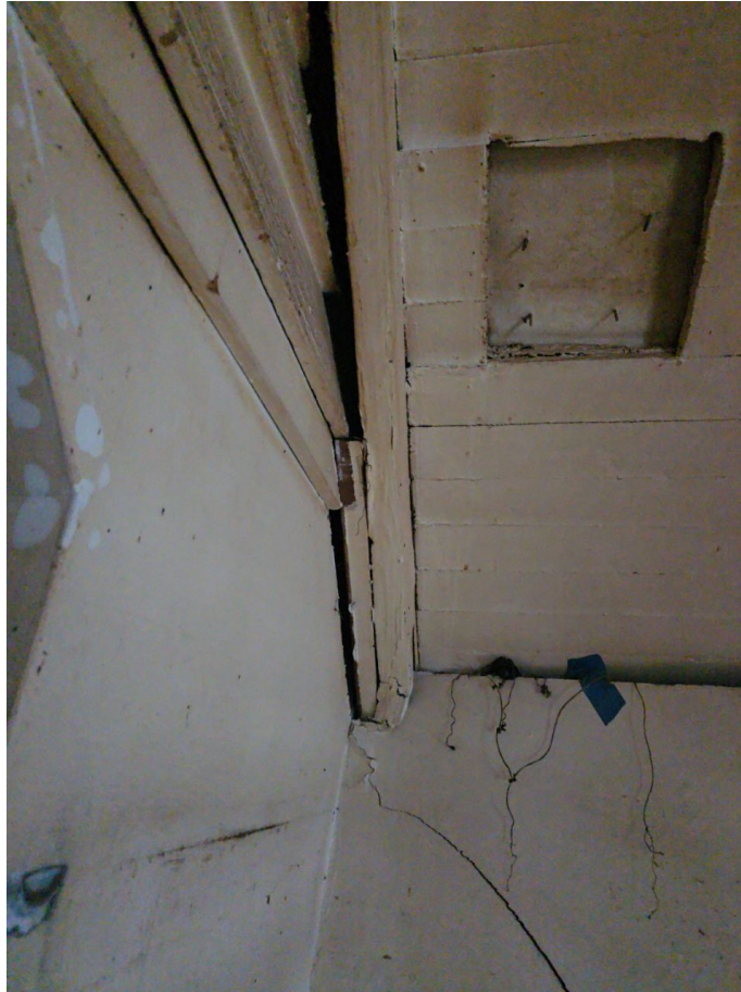
SEPARATED ROOF FRAMING
