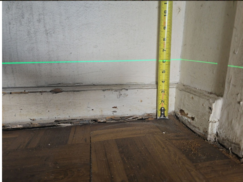
UNLEVEL FLOOR (SUNKEN FOUNDATION & FRAMING)
