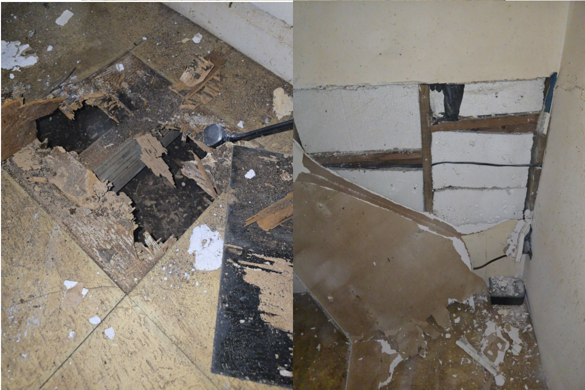
DETERIORATED FLOOR FRAMING & SHEATHING
