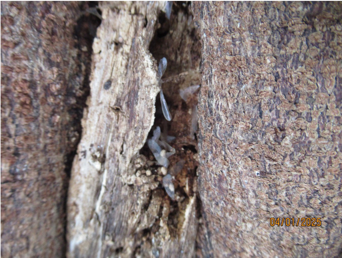
2 photos showing termites and their damage resulting in decay
