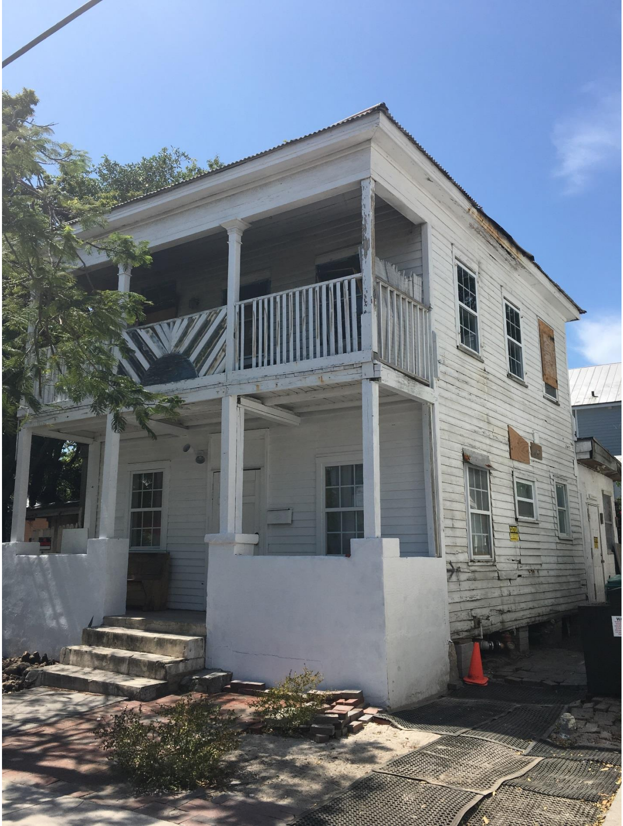
221 Petronia Street, Key West, Florida 33040 SITE VISIT – 3/31/2016
