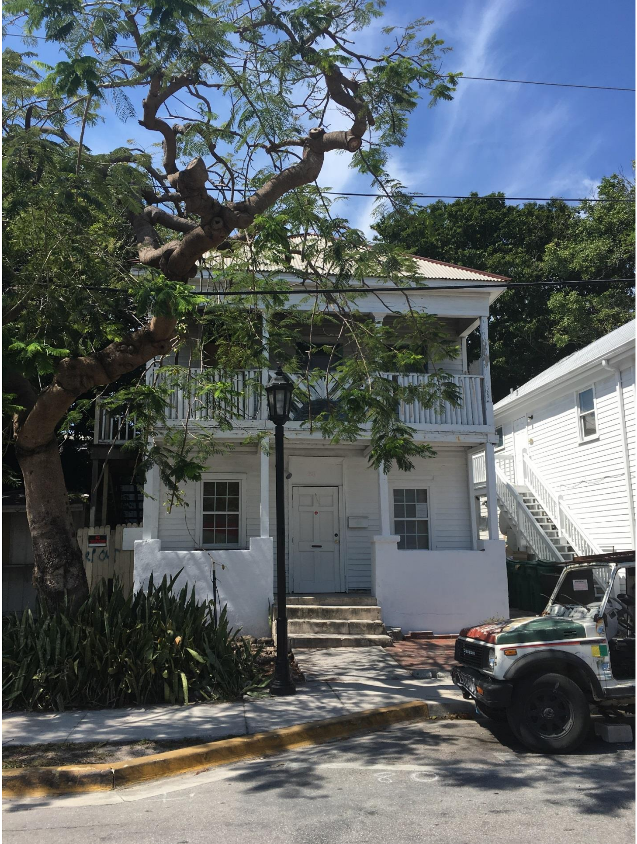
221 Petronia Street, Key West, Florida 33040 SITE VISIT – 3/31/2016
