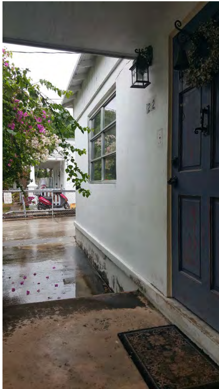
1212 Margaret Street – View from Rear Illustrating Former Front Porch with Stucco Façade
