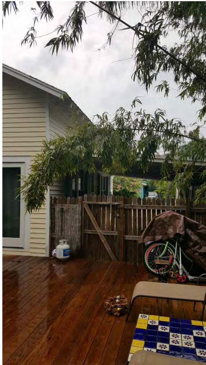
1212 Margaret Street – View from Rear Illustrating Carport
