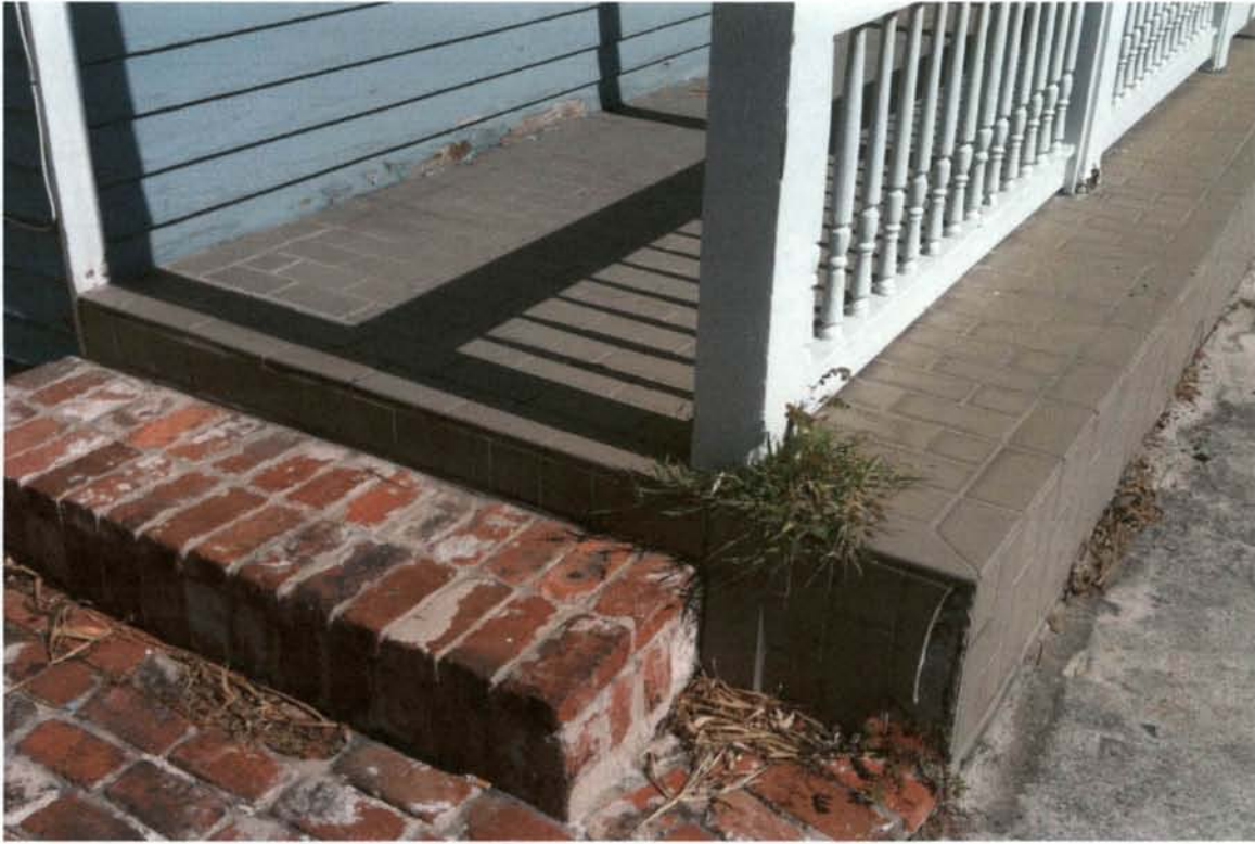
FRONT PORCH FLOOR
