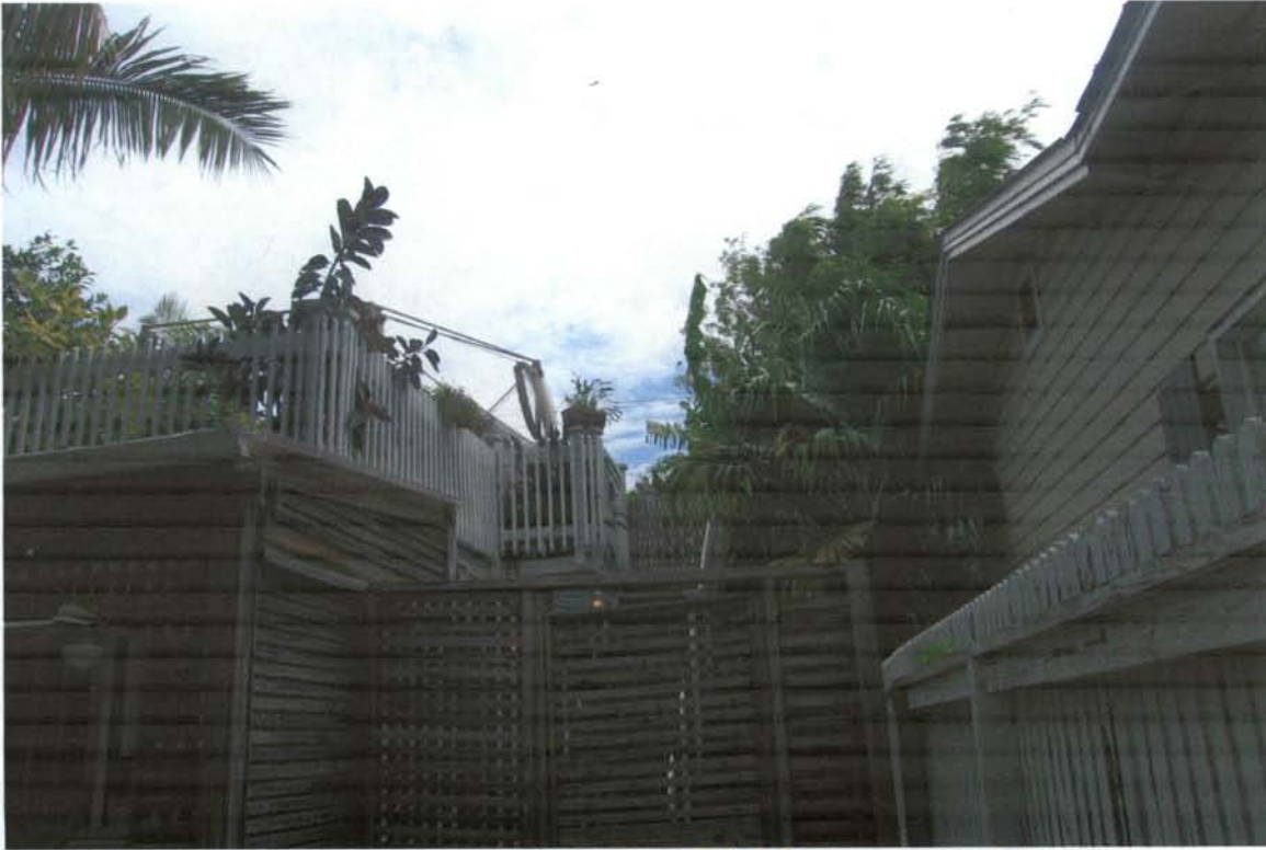
REAR, 2 ND FLOOR DECK
